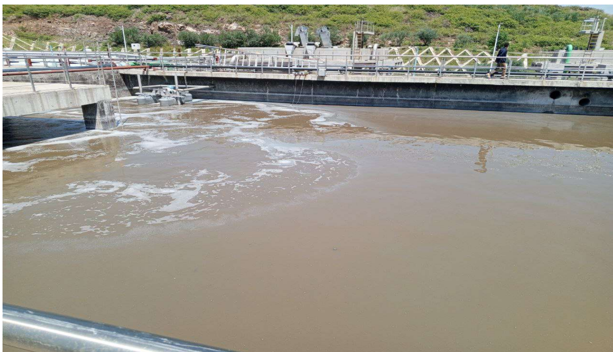
Figure 5: Sampling point in Adama Industrial Park ZLD plant (Equalization tank B)
