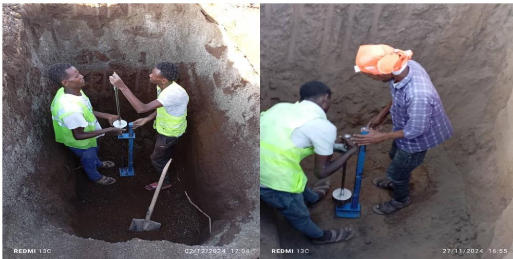
Figure 3-15 Dynamic Cone Penetrometer (DCP) Test
