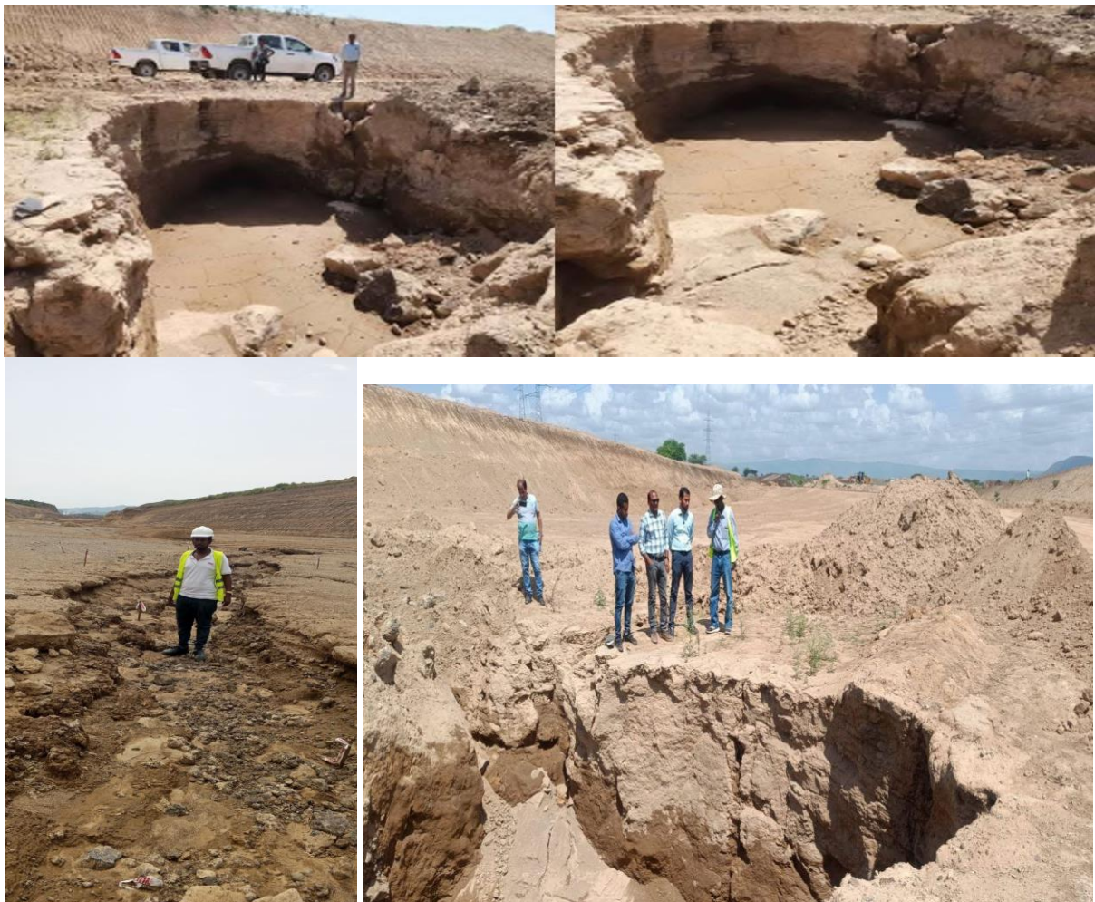
Figure 3-8: Representative pictures for potential Void Zone at km25
