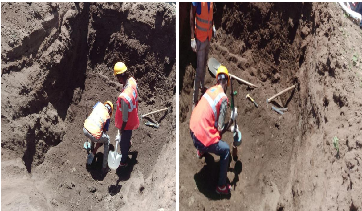
Figure 3.9 excavation and shield tube
