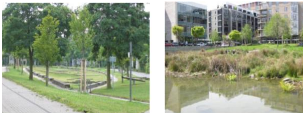
FIGURE 2.5: DETENTION POND (DRY) AND (WET) TANNER SPRINGS PARK, USA
