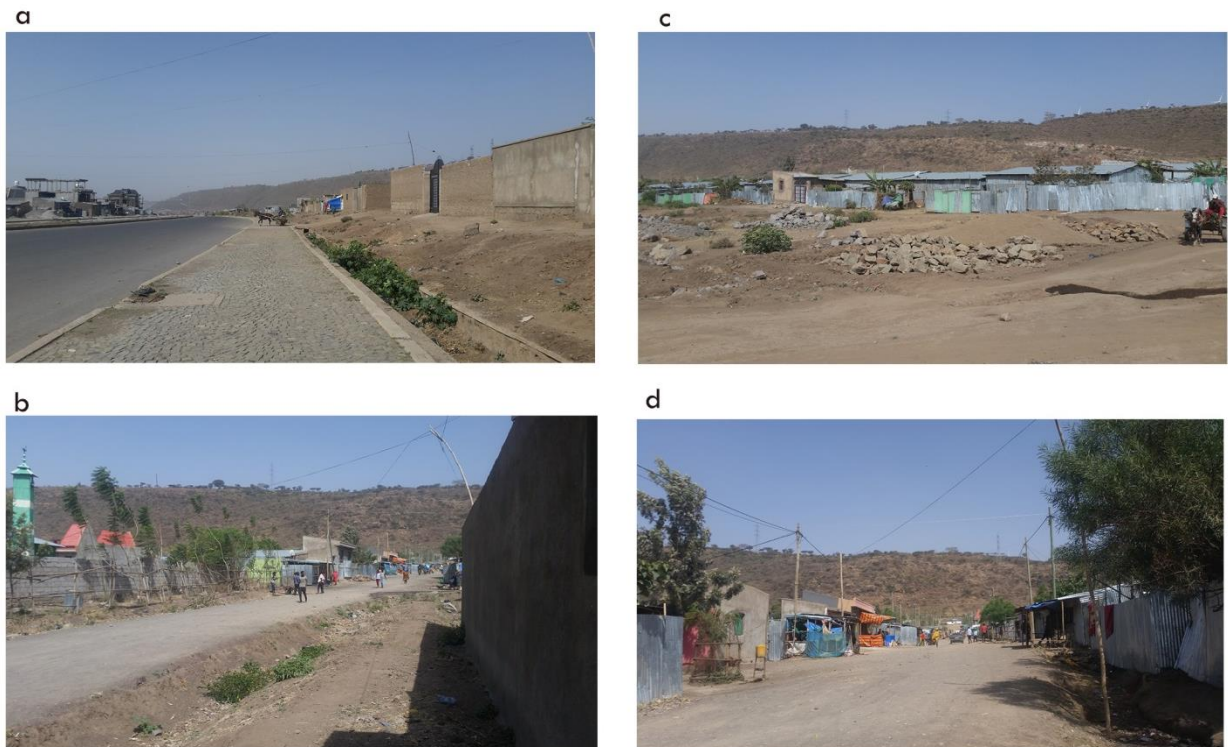
Figure 22: Pictures from site three. Main road in front of the site (a), the only road connects the neighborhood to the main road (b), neighborhood streets(c &d).
