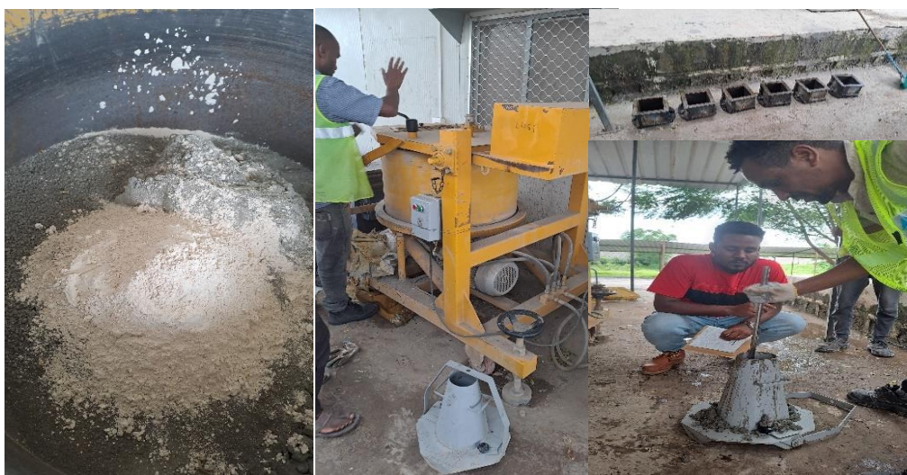
Figure 10 Concrete batching and specimen preparation.
