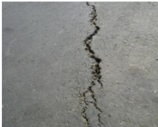
Figure 4: Longitudinal crack
