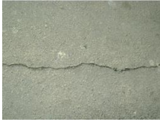
Figure 5: Transverse Crack
