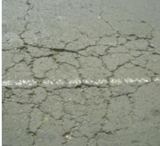
Figure 2: Alligator crack
