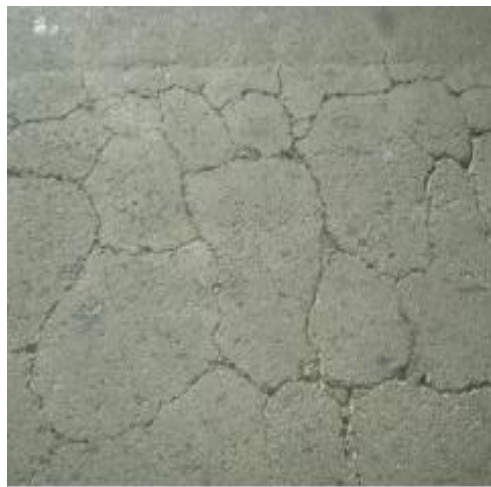
Figure 3: Block crack
