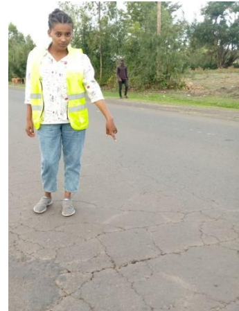
Block crack
