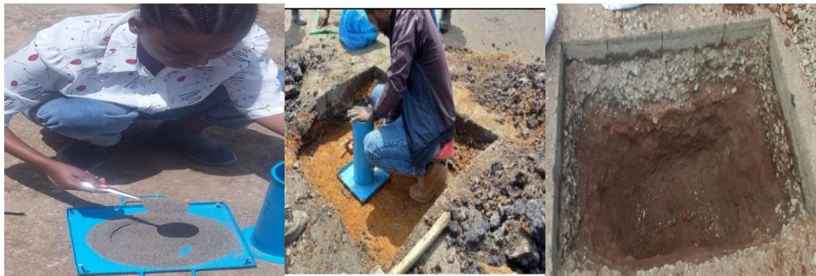
Figure 16: Field density test and pit after sampling at Km 9+580 and 6+230
