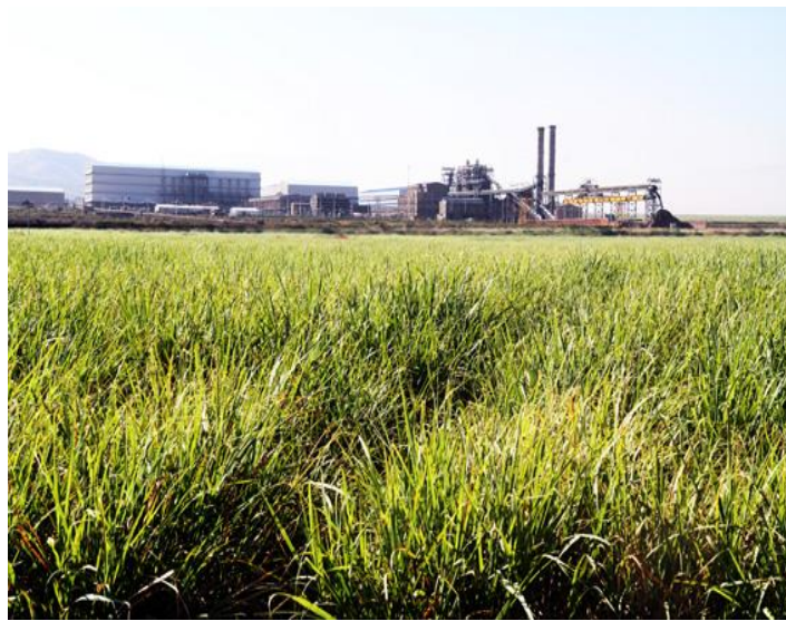
Figure 1. 1. Partial view of Wonji/ Shoa Sugar Factory
