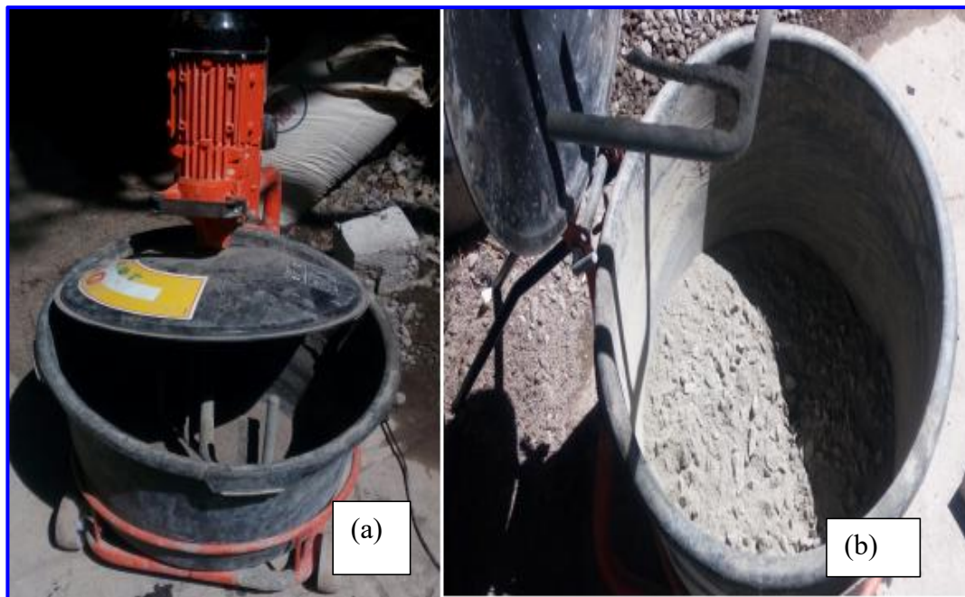
Figure 3.10 Concrete Mixing: Mixer (a), Dry Mix (b)
