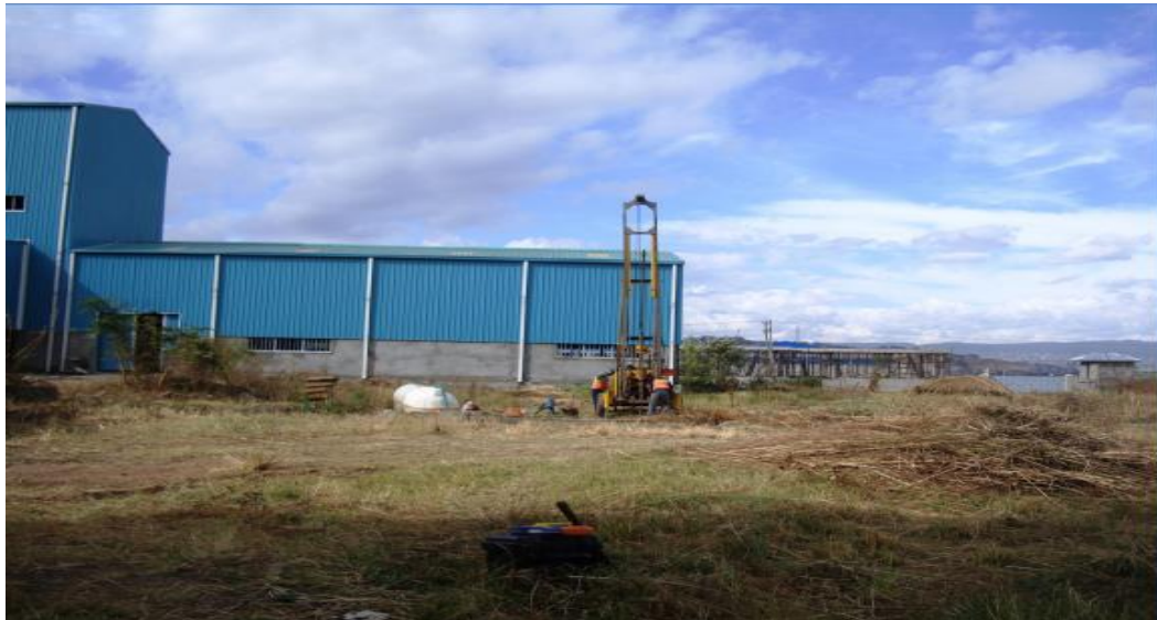
Figure 3.2 Partial view of the proposed Effluent Treatment Plant site.
