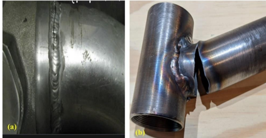
Figure 1.2. Weld bead specimens defect detected from the Asella Malt plant firm: (a) Weld bead crack and Base metal HAZ crack (from the industry).
