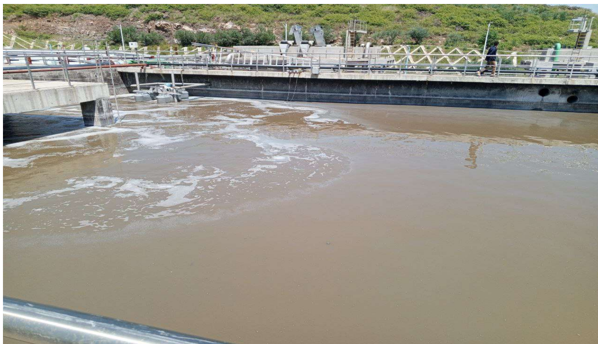
Figure 3. Sampling unit in Adama Industrial Park ZLD plant (Equalization tank A)
