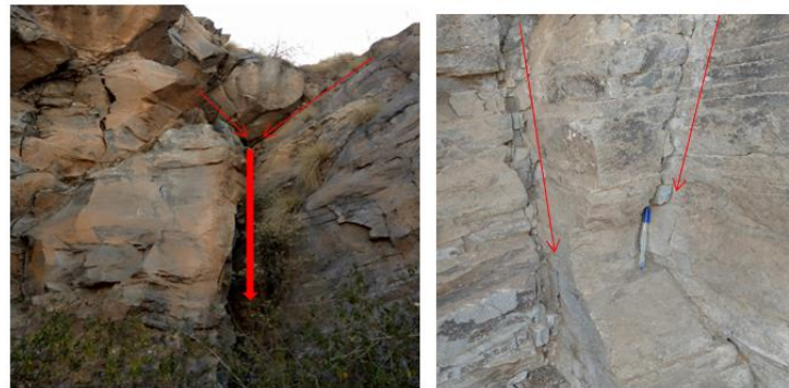
Fig 4.6: Field photos of Joints (wedge failure forming joints at left).
