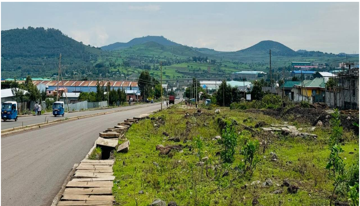
Industrial land use and vacant open space for greenery.
