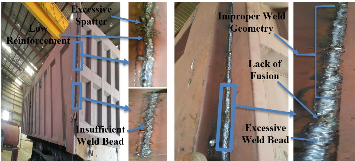
Figure 1.2: Weld defects and imperfections (Mesfine Industrial Engineering, Ethiopia)
