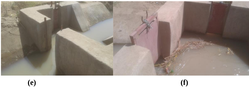
Figure 4.2. Current status of Division box (November 12/2017)
