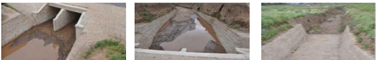
Figure 4.32: Photo of two drainage canals diverted to Migira from Expressway
