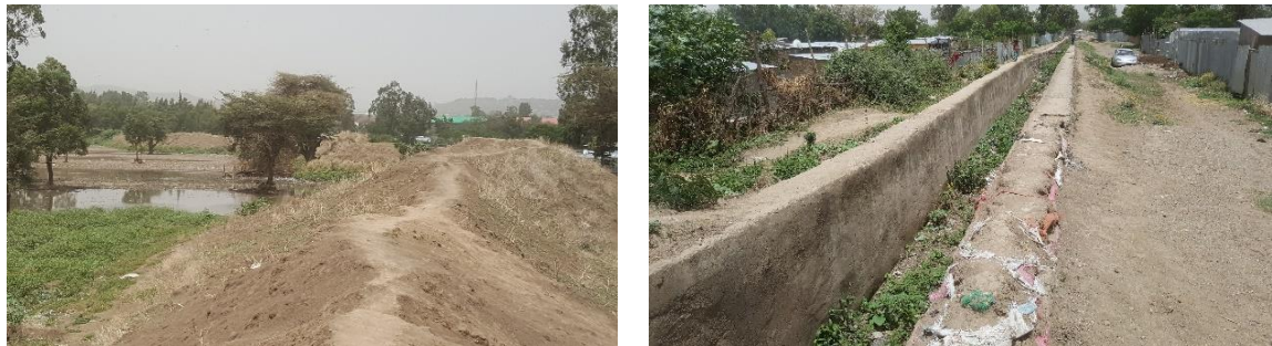
Figure 4.26: Photo of access roads and liquid waste drainage line in Migira Pond area
