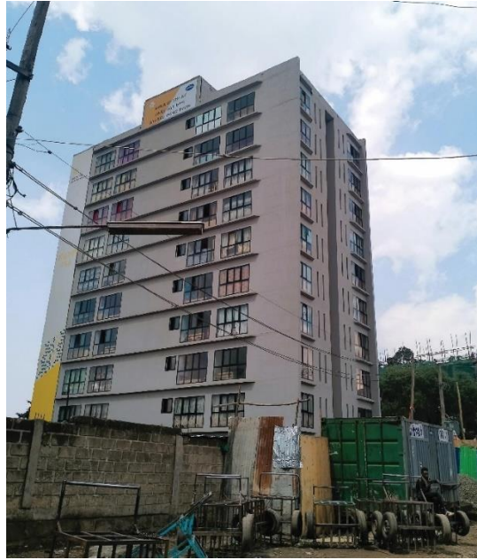
Figure 2.2: Riche PPP Housing (Source: researcher, 2024)
