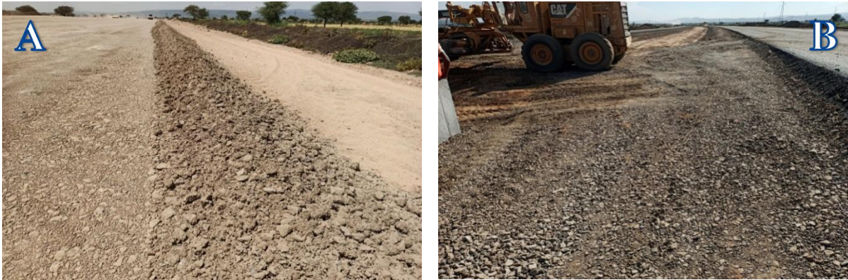
Figure 4.5 Wastes on Sub Base Layer work
