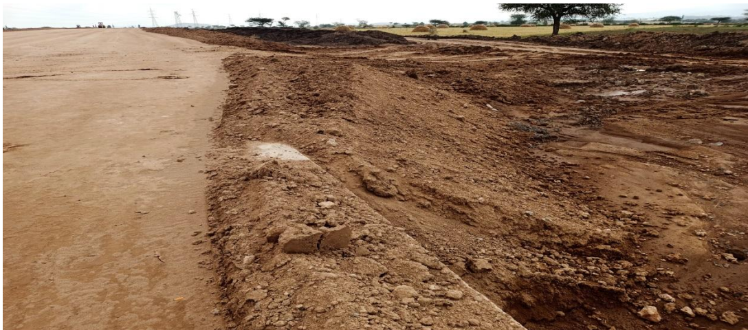
Fig 4 Removed excess material from the site
