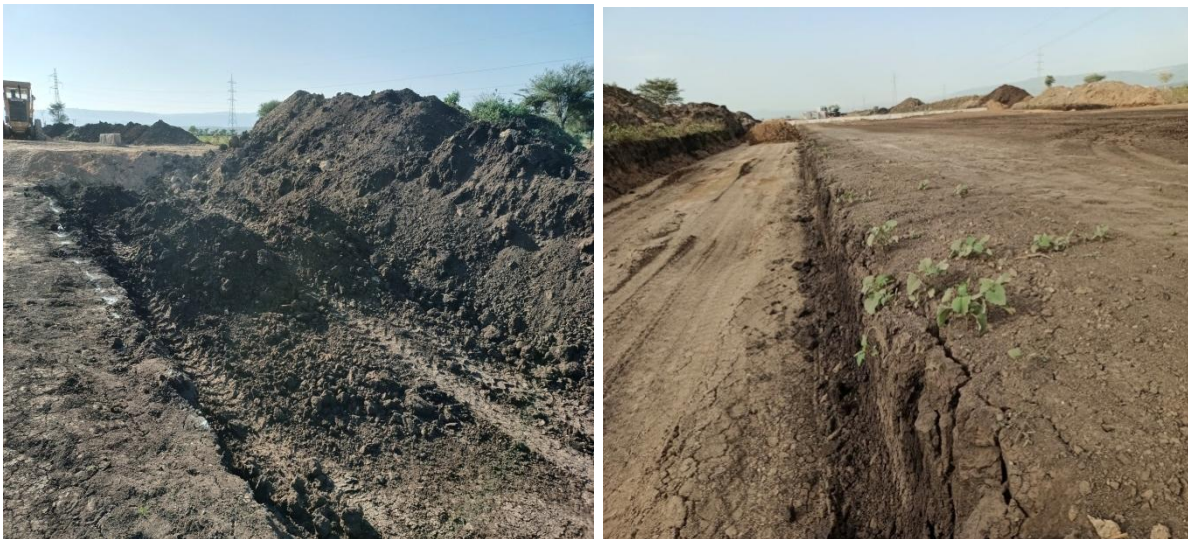
Fig 2 Rework of Road Bed and Undercut Replacement
