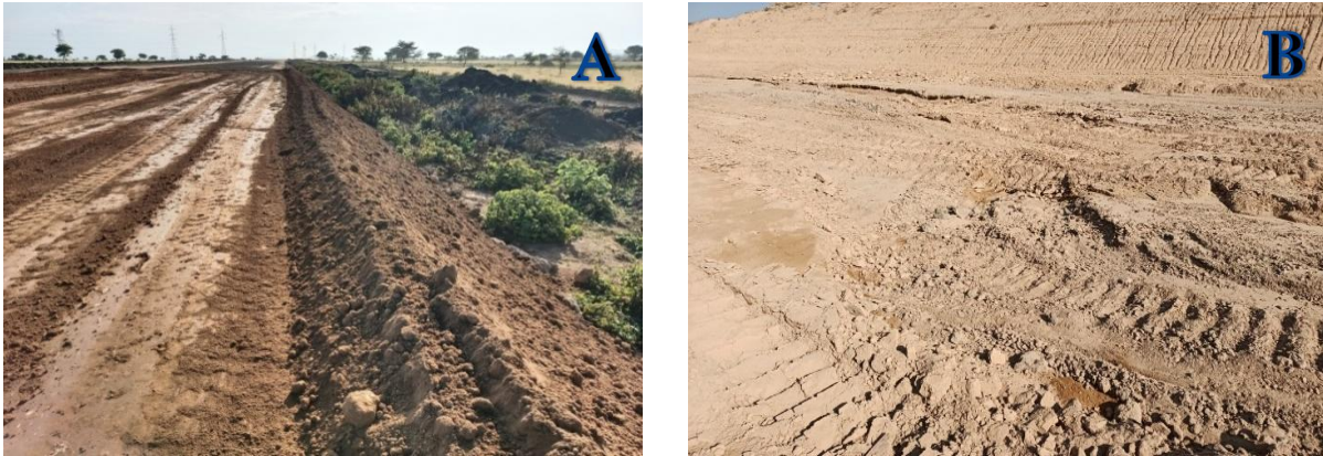
Figure 4.4 Wastes on Embankment Layer work
