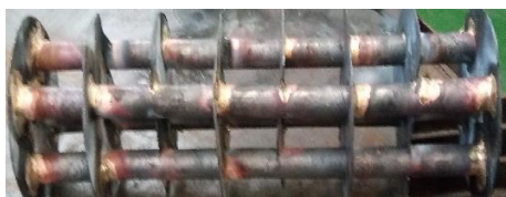
Welding of baffles and tubes
