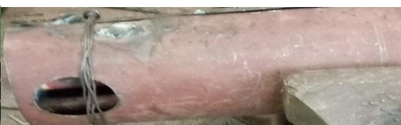
Covering the central part by shell
