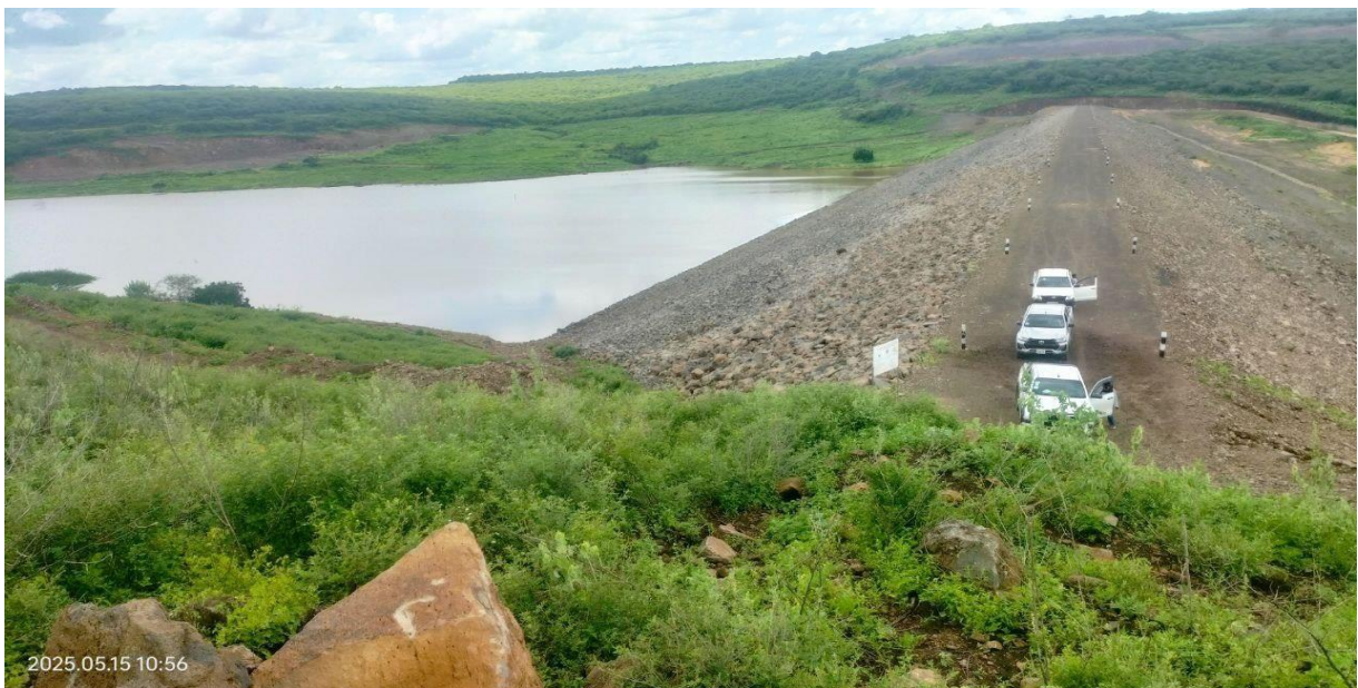
Appendix Figure 7-2: Upstream of the dam
