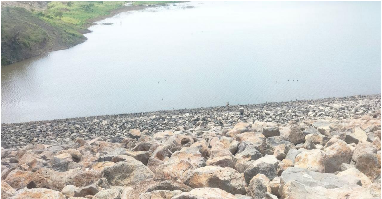
Appendix Figure 7-1: The dam store of water
