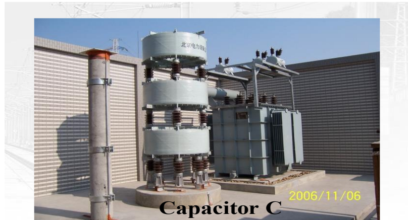
Figure 3.62 Capacitance compensation device
