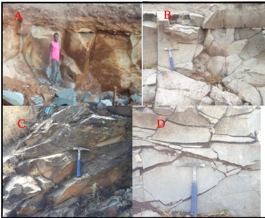
Figure 22 Different joint sets a) in reservoir area b) on the right abutment c and d) on the left abutment.
