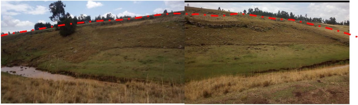
Figure 50 Unstable slope section in the reservoir area RRSS1.
