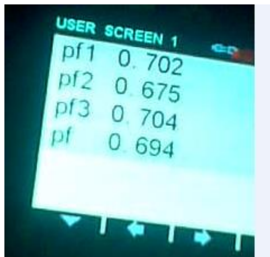
Figure A4 . Transformer2 1mva Transformer Load Power Factor Profile Displayed on Power Stability Recorder
