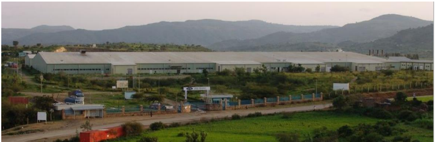
Figure 1.6 Part of Almeda Textile Factory
