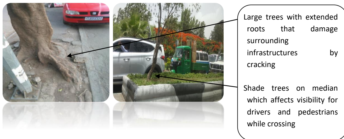
Figure 28: Green infrastructure provision in the case site
