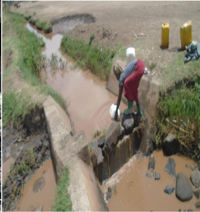
using stone to divert water to intake
