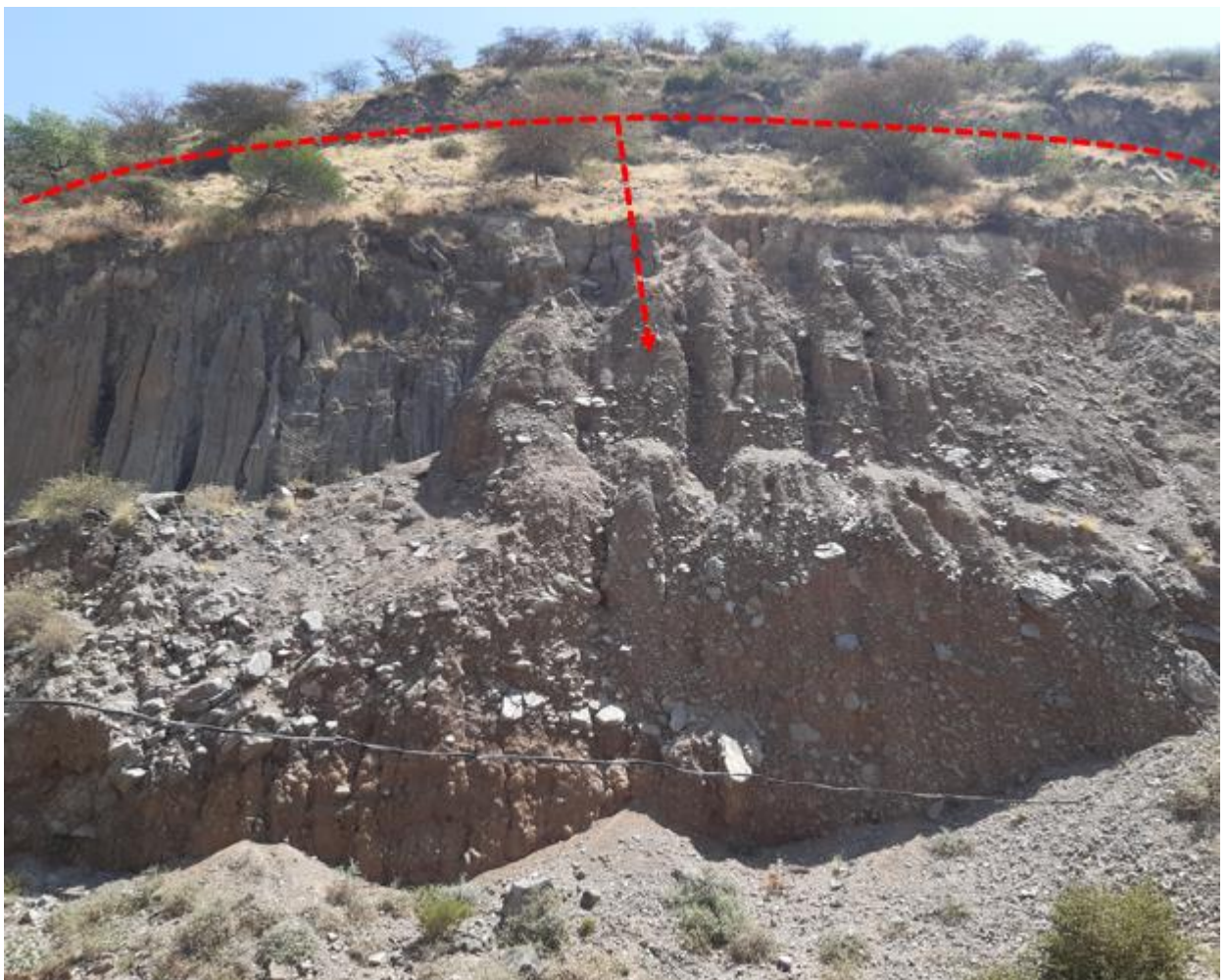
Figure 5. 12 Existing field condition of slope section SS3.
