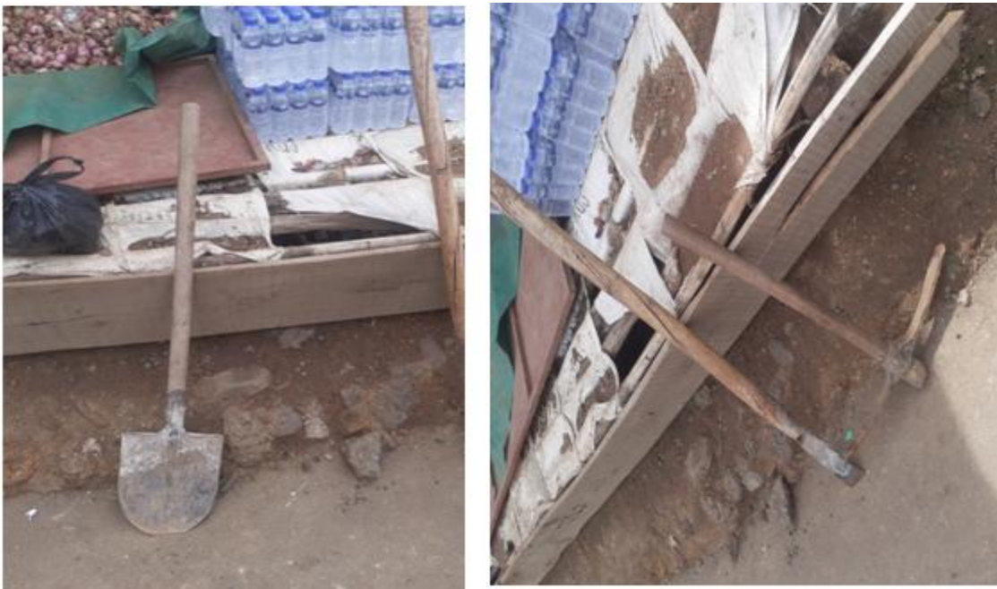
Figure 3.4: Traditional excavation equipment's used for excavation
