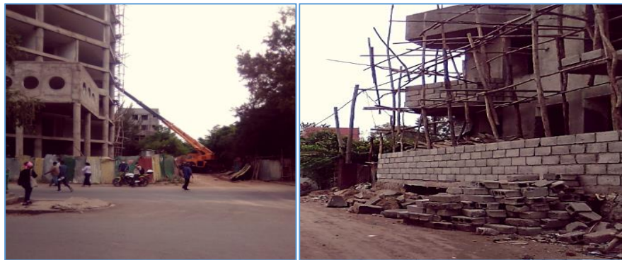
Figure 4.16. Accessibility problems around under-construction buildings (Field survey, 2020).
