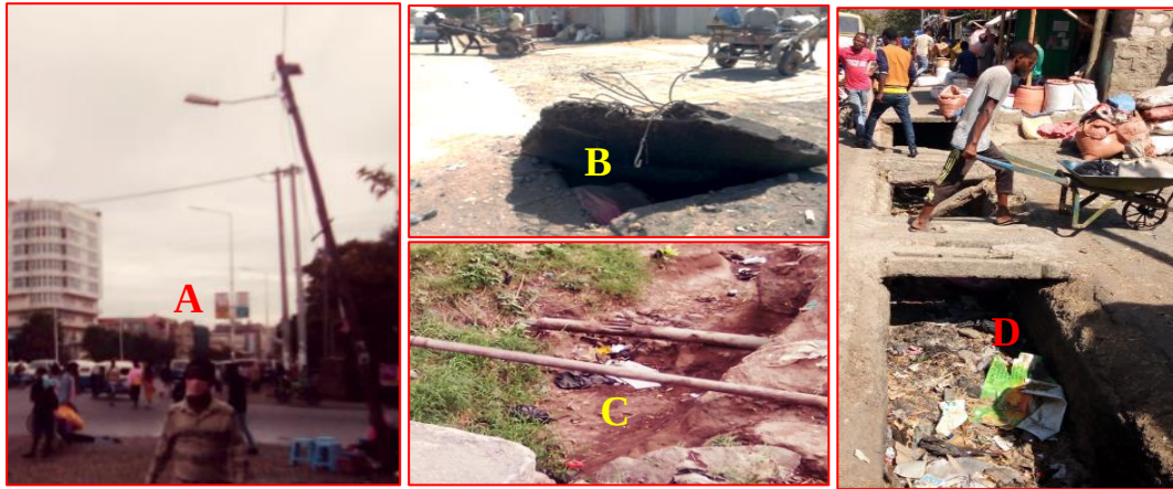
Figure 4.4. Problems in utility lines (Field survey, 2020).
