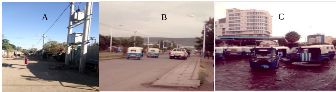
Figure 4.41. Utility and Infrastructures problems (Field survey, 2020).
