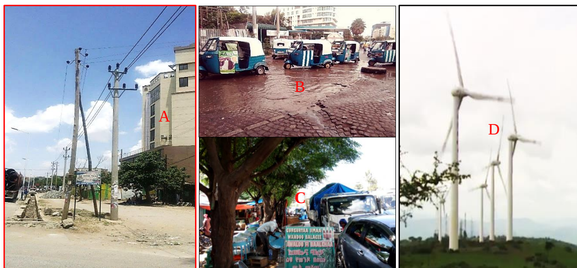
Figure 4.52. Problems of capital web & lack of efficiency & adaptability (Field survey, 2020).
