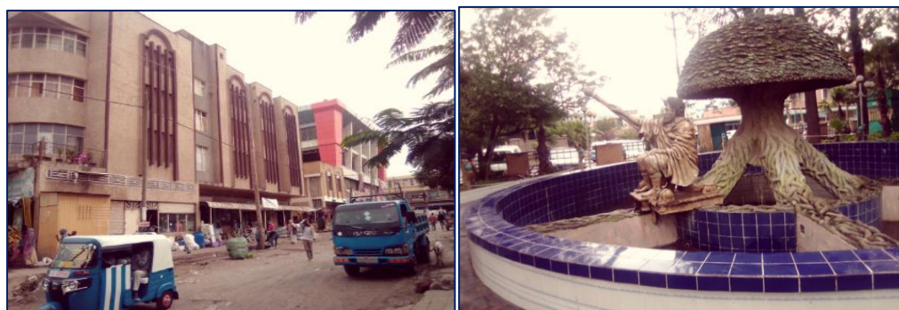
Figure 4.47. Some building facade treatments & Abba Gadaa statue. (Field survey, 2020).
