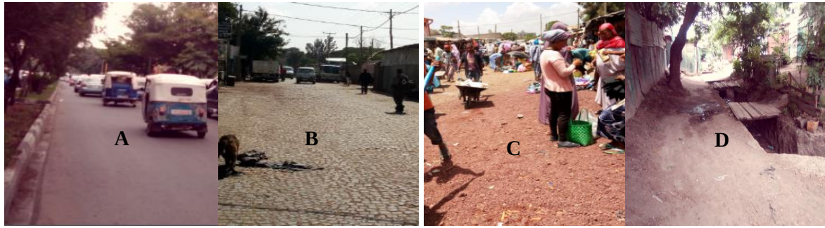
Figure 4.34. Problems of street finishing materials (Field survey, 2020).
