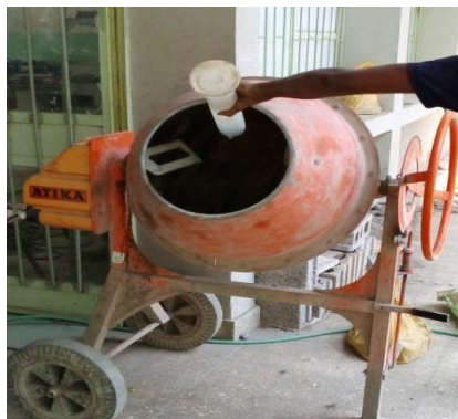
A. Mixing concrete ingredients by Mixer
