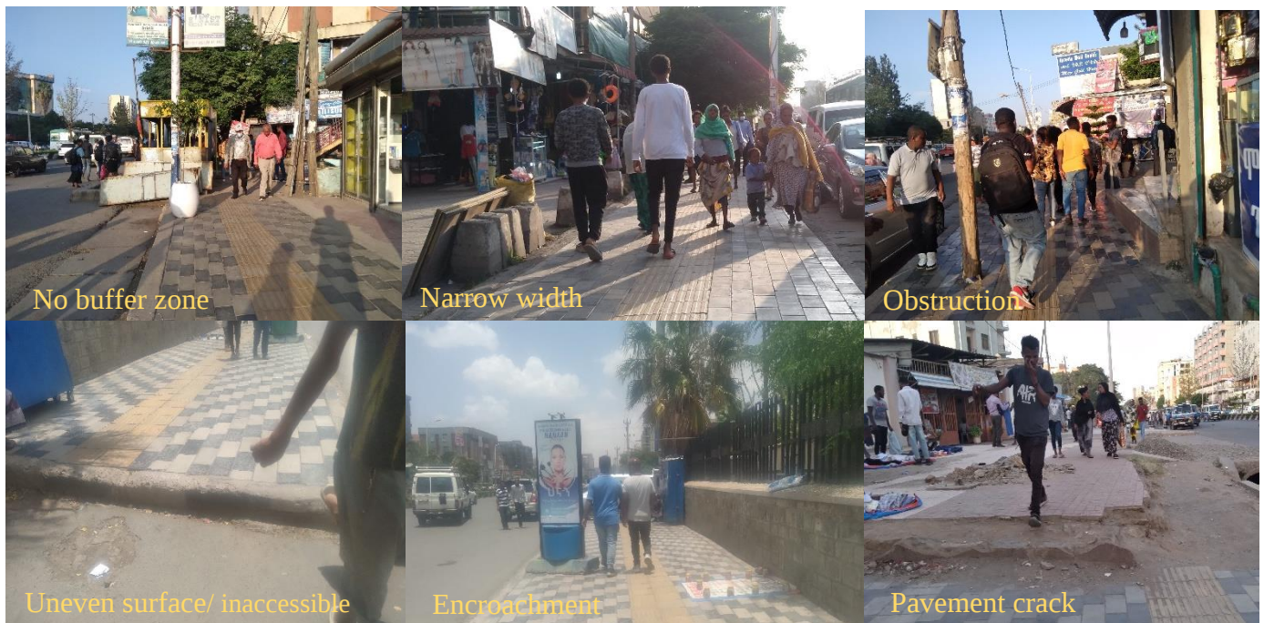
Figure 4-1: Franko segment sidewalk physical condition (source: Author site observation)
