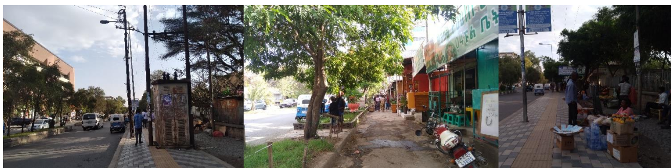
Figure 4-3: 04 - Mariam church segment sidewalk physical condition
