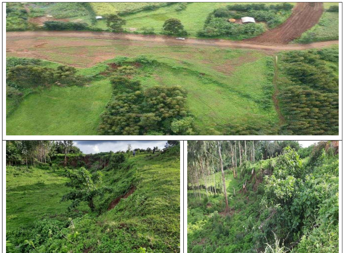
Figure 4.5: Landslide movement from station 67+500 – km 67+570
