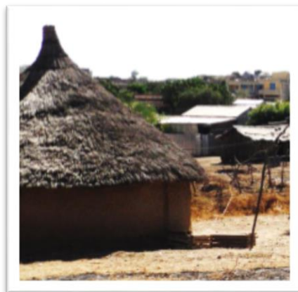
Figure 24 Roof shaded wall (field work,2020)
