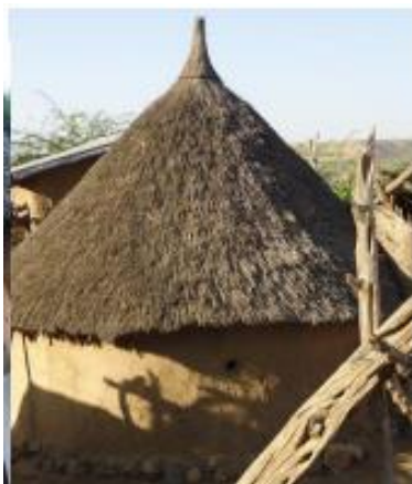
Figure 24 Roof shaded wall (field work,2020)
