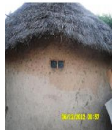
Figure 23 Narrow windows (field work,2020)
