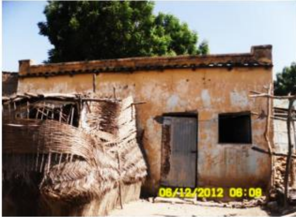
Figure 16 Old thick brick houses with basket shelter extension (field work,2020)
