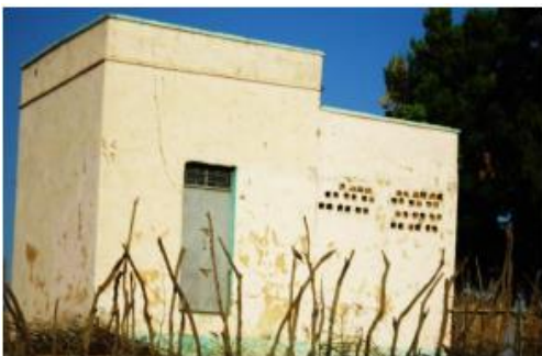
Figure 19 White painted external wall (field work,2020)
