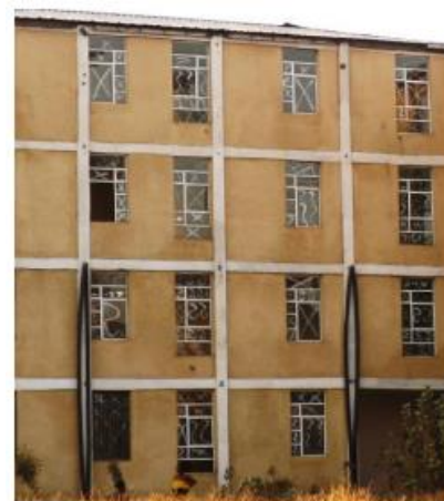
Figure 31 Bended down pipes (field work,2020)
