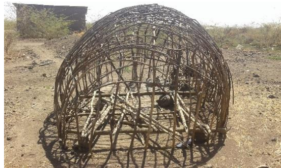
Figure 12 Movable house structure outline (field work,2020)
