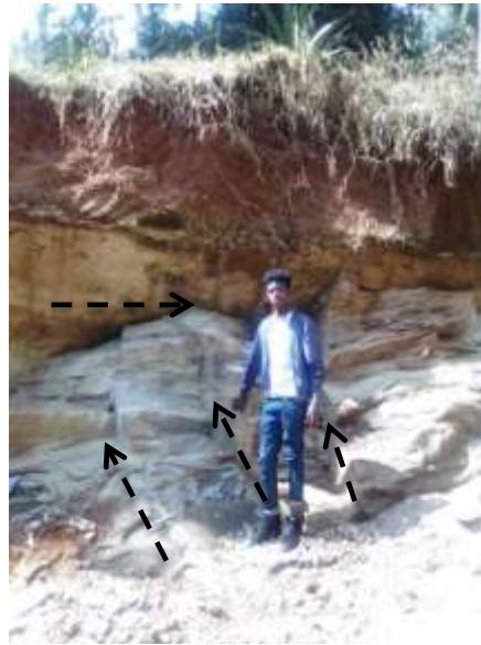
Figure1.12 Minor local fault and Joints on ignimbrite along to Hawassa route
