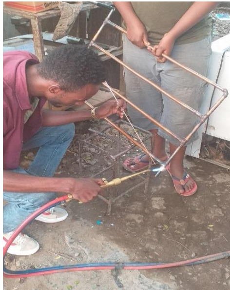
Figure 3.5 The image of welding the riser and header with elbows at joints using oxy-acetylene welding
