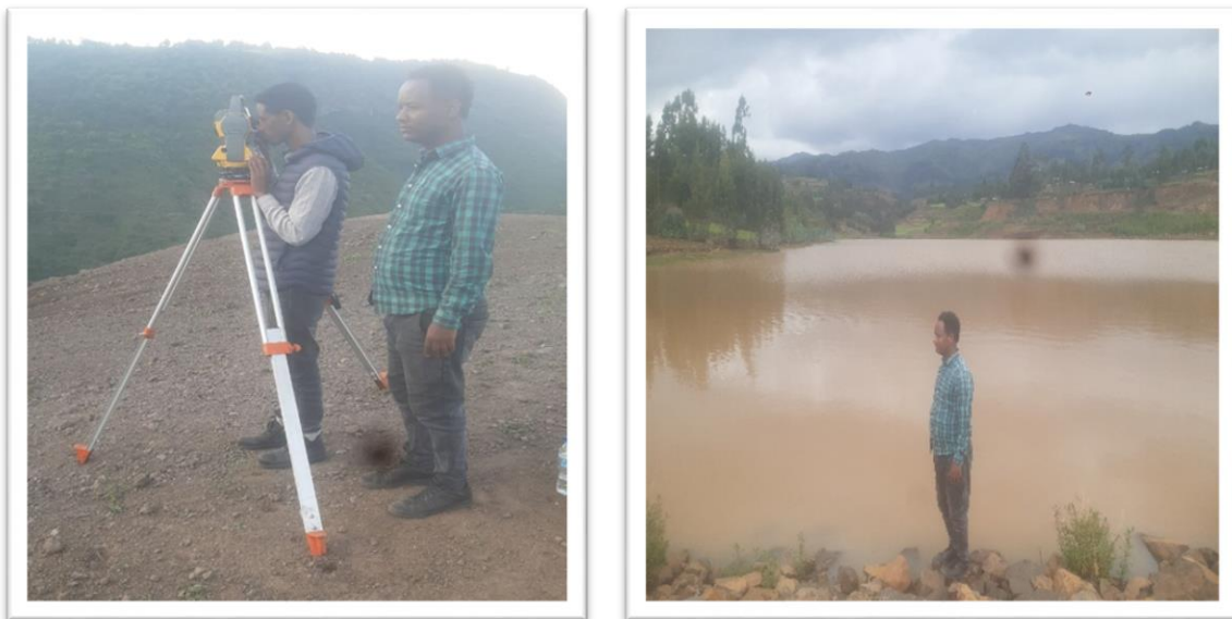
Appendix A2 Aguat Wuha Dam Crest and U/s Water Level Measurement (18/04/2023 )
