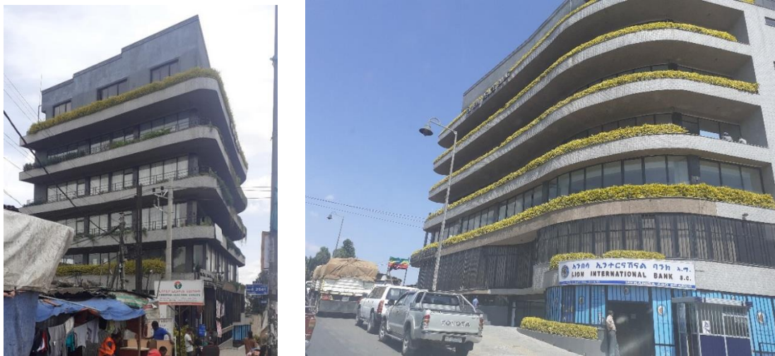
Figure 14: Peace building around Mekanisa (Source: Researcher, 2021)
