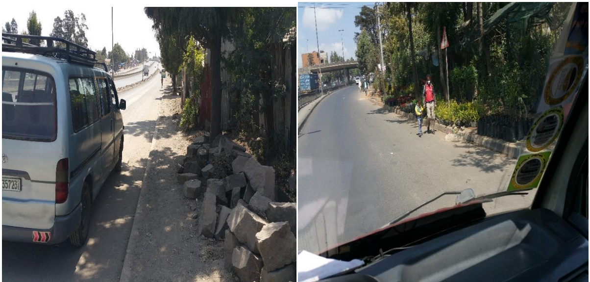
Figure 4. 55: accumulation of stone and garden trees on walkway
