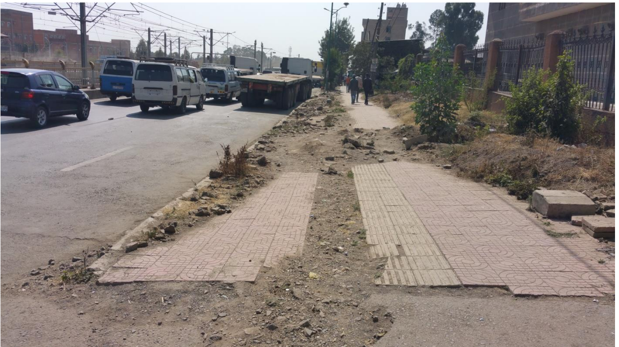
Figure 4. 77: Absence of sidewalk and inaccessible sidewalk on Mesaltegna to Adeyababa road segments
