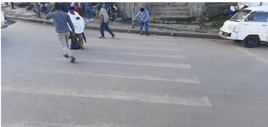
Figure 4. 22: Curb cuts with raised at zebra obstructing wheelchairs.
