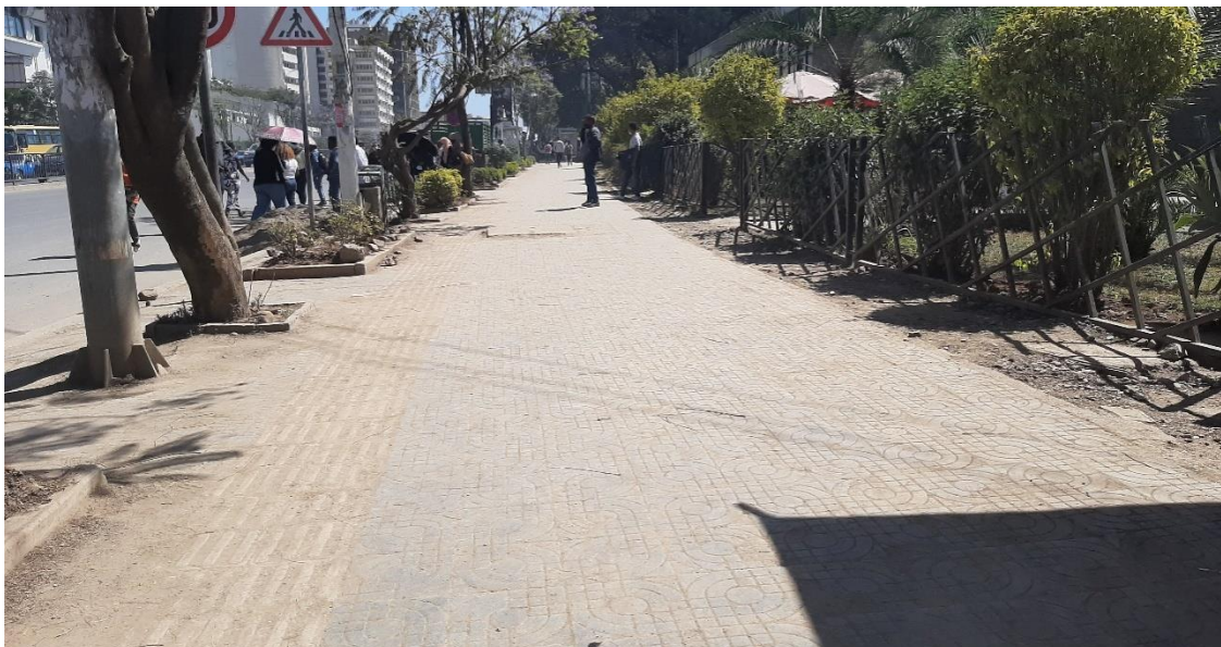
Figure 4. 15: Road barriers and improper aligned tactile surface for visual disabled
