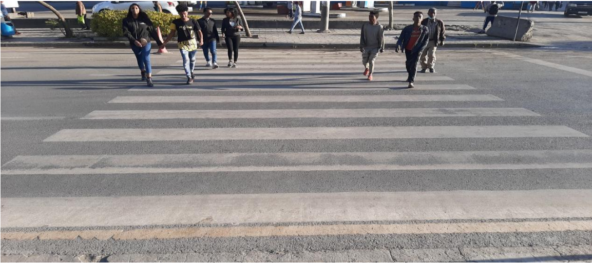
Figure 4. 33: lack ramp for wheelchair users at crossing
