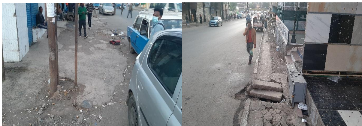
Figure 4. 64: Road barriers and narrow walkways
