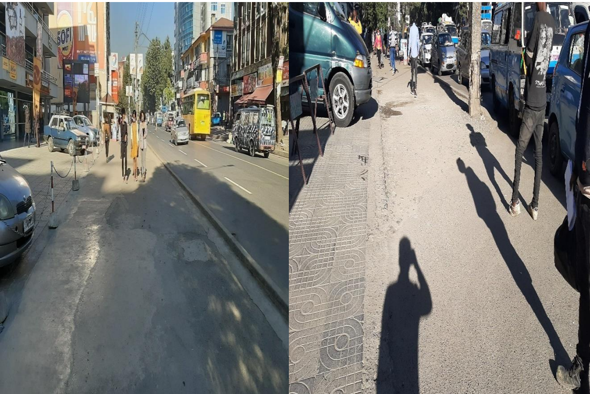
Figure 4. 59: lack of proper walkways and tactile surface for visual disabled
