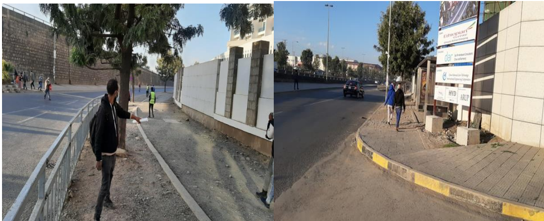
Figure 4. 31: Improper walkway, tactile surface, and unsafe for disable people
