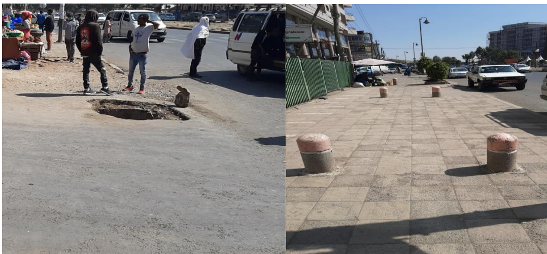
Figure 4. 10: Open Ditch and Obstacles on Walkway.
