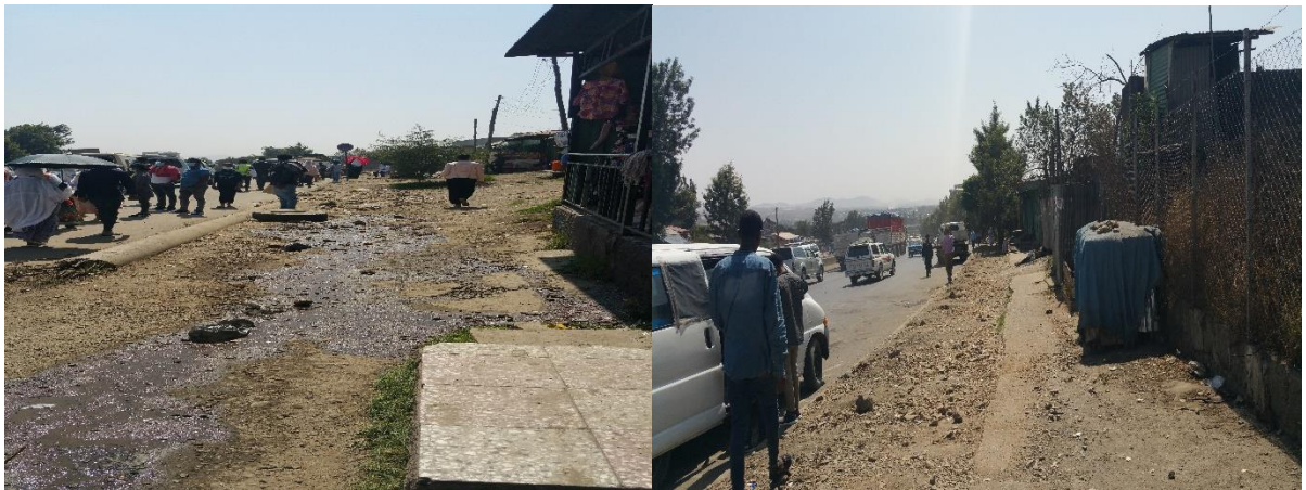
Figure 4. 53:Lack of proper walkway
