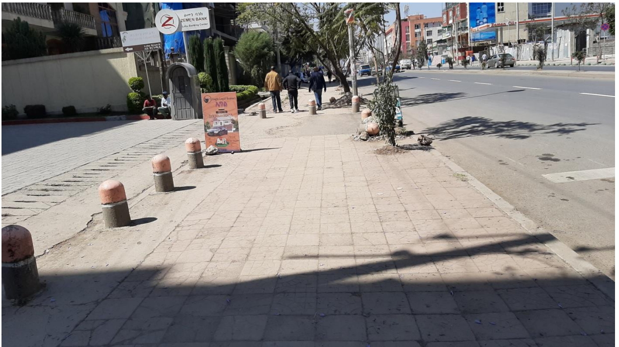
Figure 4. 82: Inaccessible routes for wheelchair users and other PwDs
