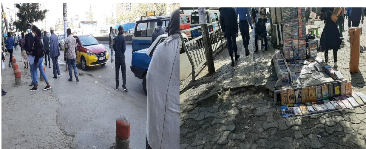
Figure 4. 65 lack of proper walkway and settled walkways
