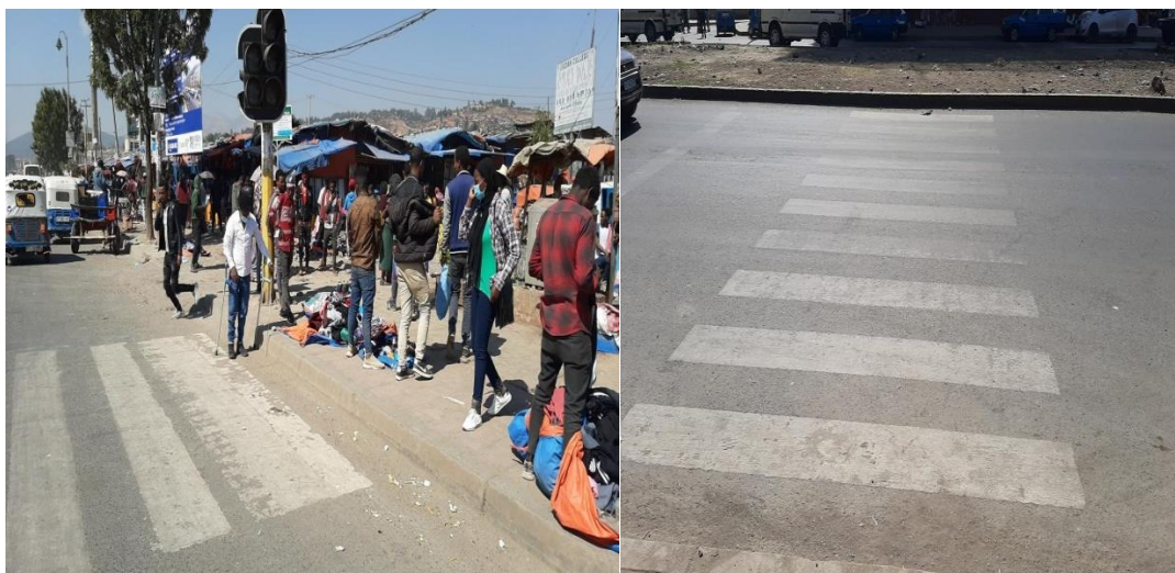
Figure 4. 8: Lack of ramp for wheelchairs users
