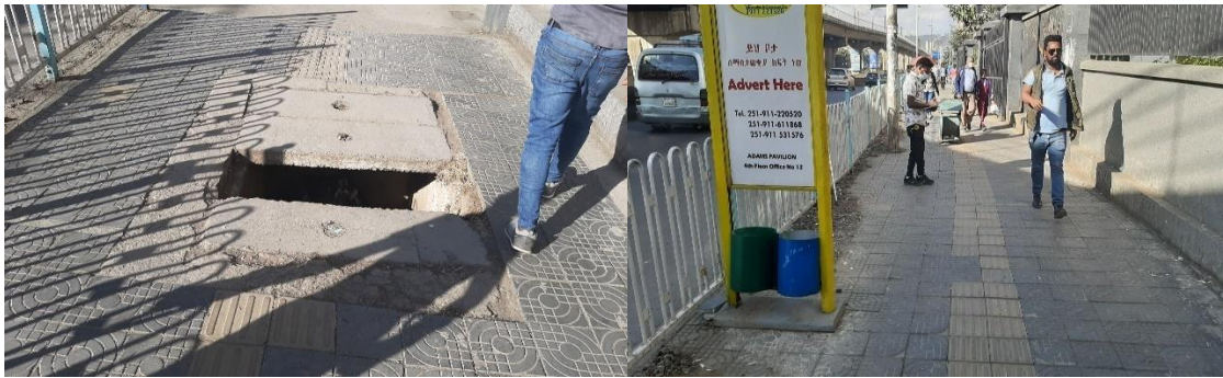
Figure 4. 40:Open ditch and road barriers on walkway
