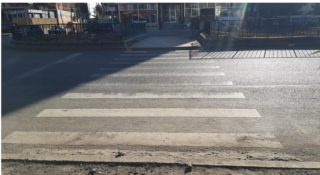
Figure 4. 43:raised edge at crossing which is not comfort to wheelchair users
