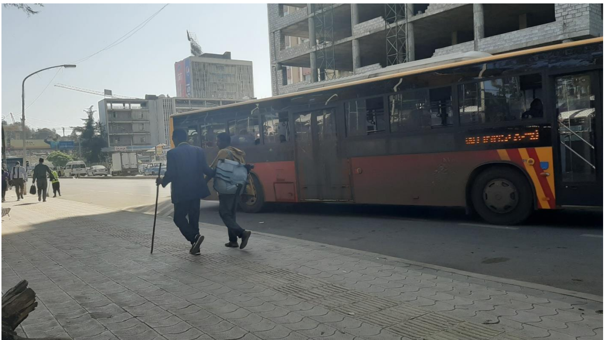
Figure 4. 76: Absence of curb ramp and tactile surface to Minilik square at Arada sub city.
