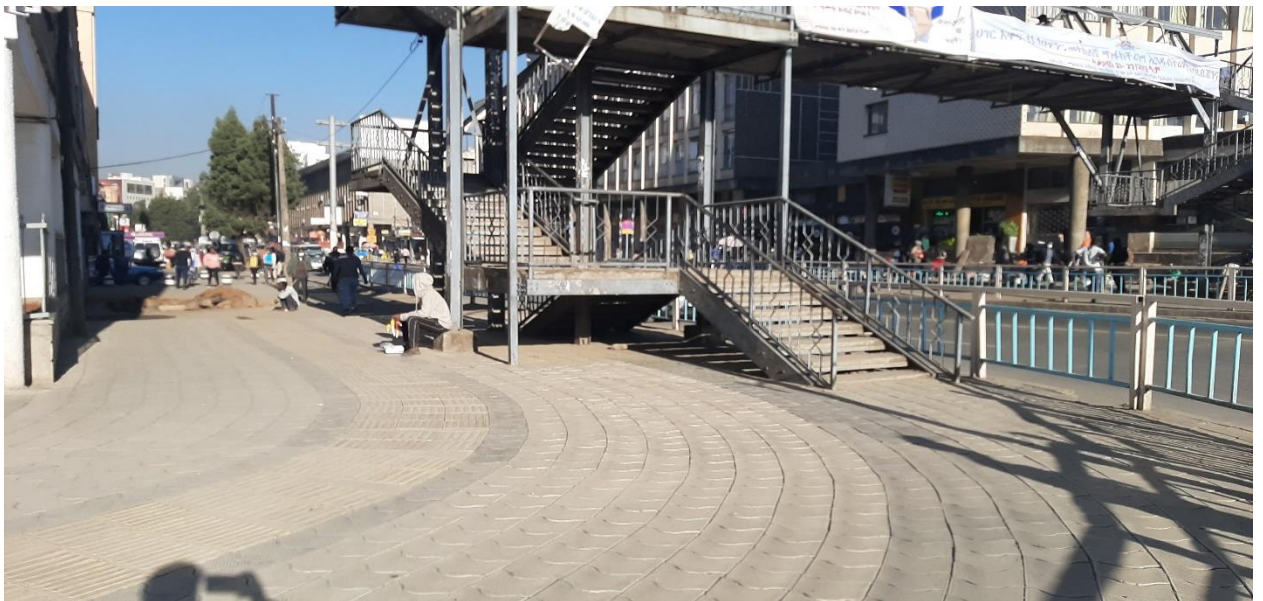
Figure 4. 57:lack of ramp for wheelchair users
