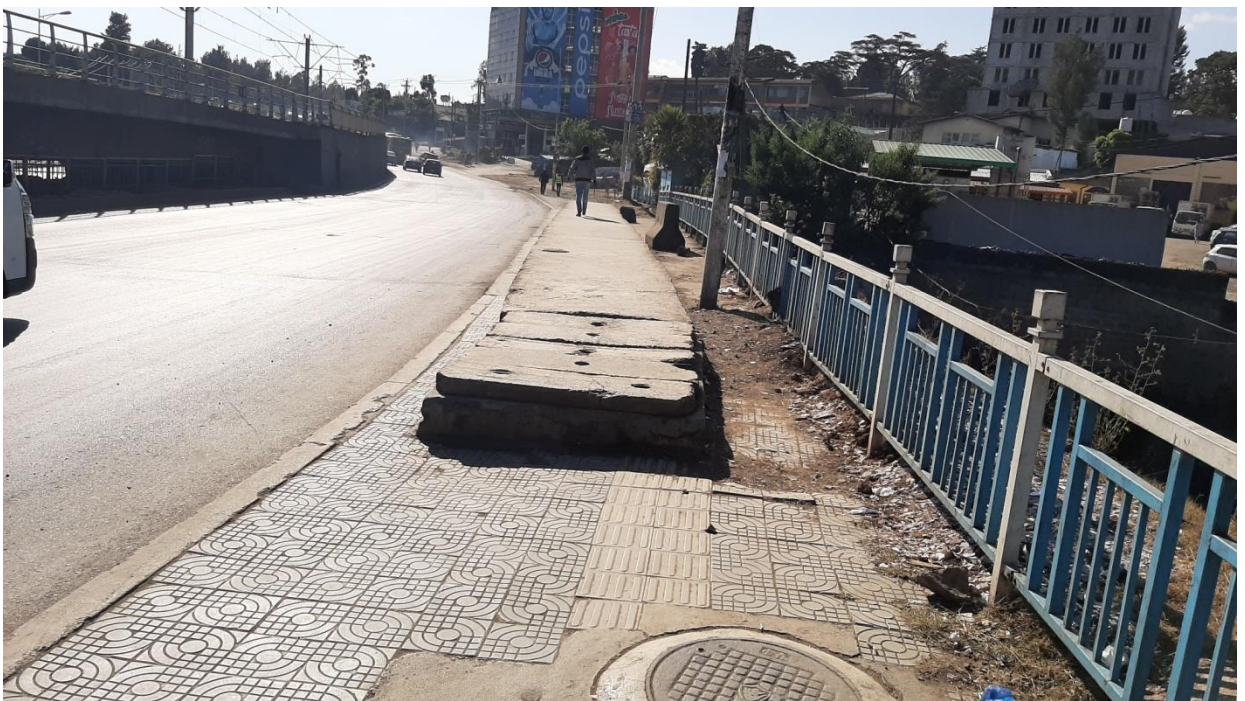
Figure 4. 80: Trees, poles and inappropriate raised sidewalks from lideta to Tor hailoch Adebabyi
