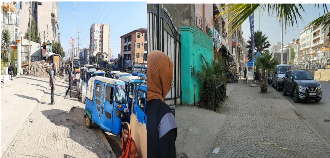
Figure 4. 42: pop out coble road and obstacles on walkways
