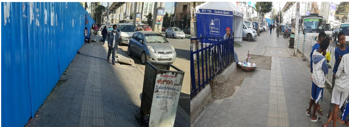
Figure 4. 41:Construction fence on walkway and dismantled walkway tile
