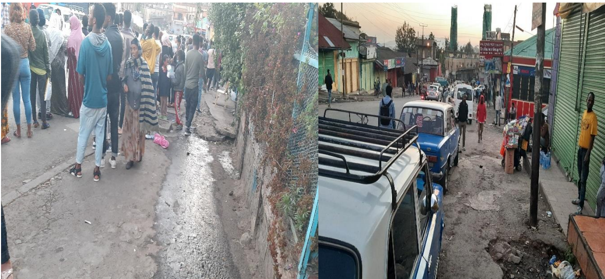
Figure 4. 63:lack of proper walkways
