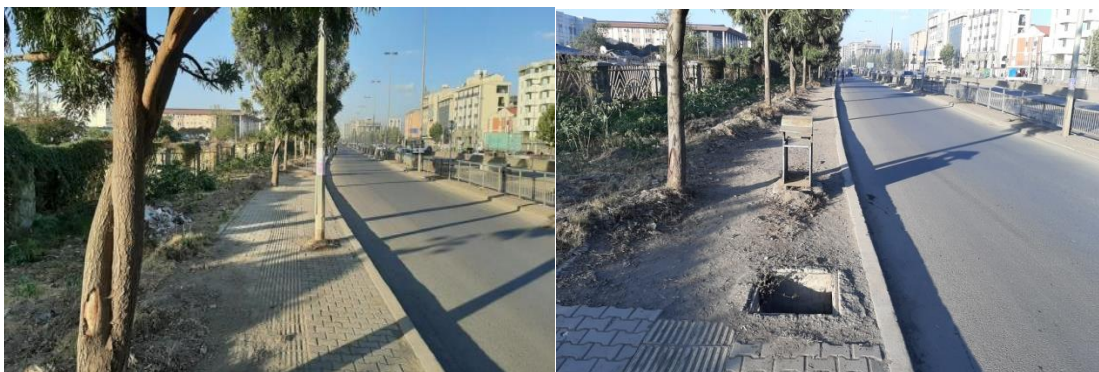
Figure 4. 32: Road barriers (trees and telephone poles) and open ditches
