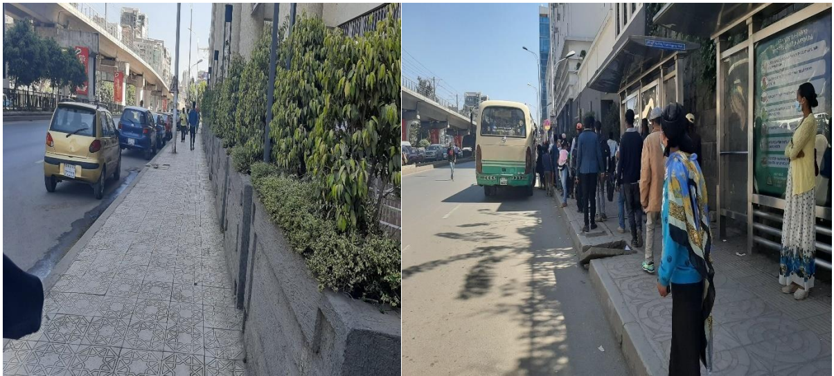
Figure 4. 14: No tactile surface for visual disability and open ditch on pedestrian way
