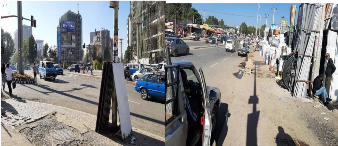
Figure 4. 36: Cracked walkways and storage of materials on walkways and lack of proper drainage
