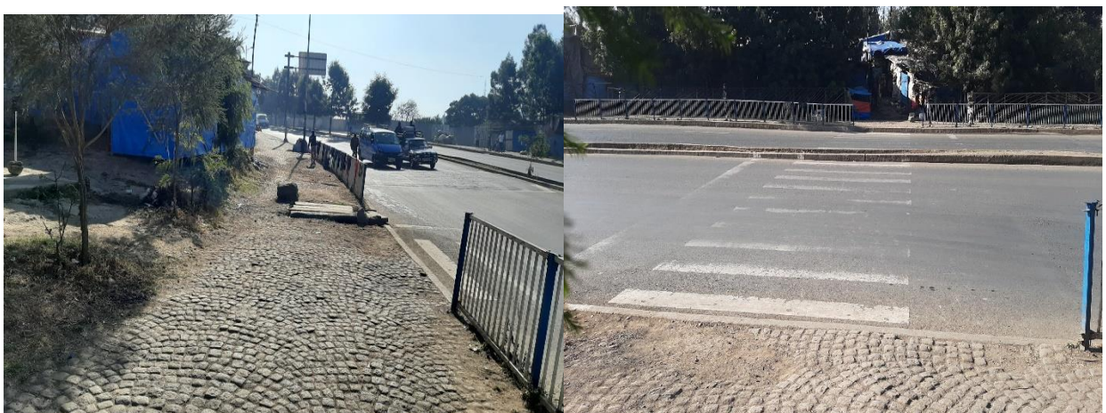
Figure 4. 46: Obstacles on walkways and raised edge at zebra
