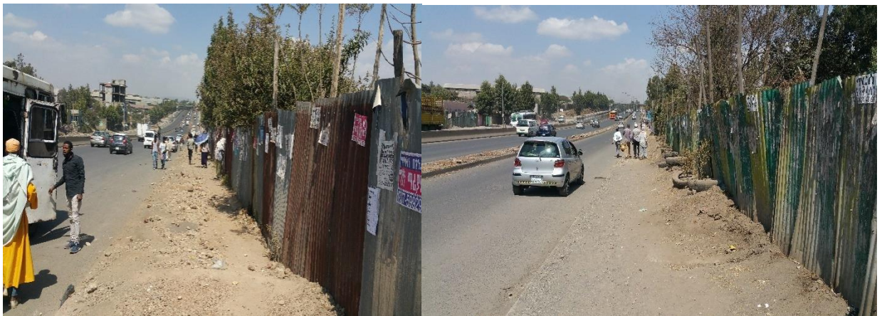
Figure 4. 54: improper walkways for disabled
