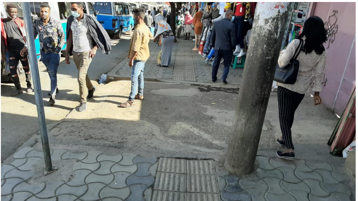
Figure 4. 79: Pavement Curb cuts without ramps and unsecured tactile surface for visual impaired from Adisu Gebeya to Chilot Adebabyi in Gulele Subcity
