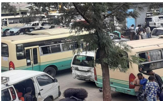
Figure 4.20: improper taxi/bus terminal space design
