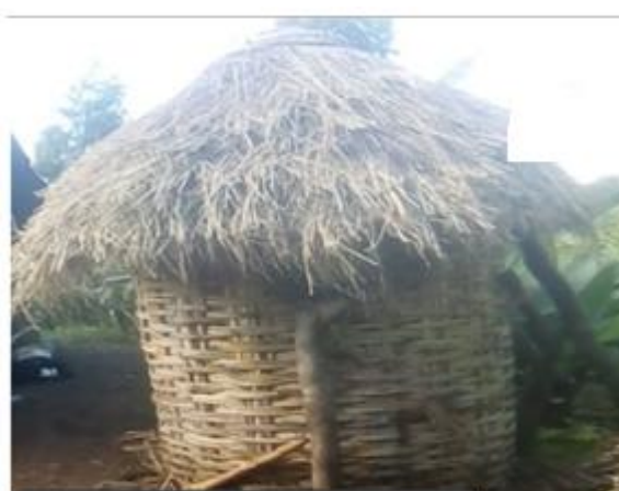
Riqa made of bamboo with a thatched grass roof
