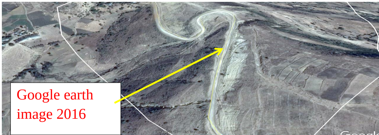
Figure 4.11(b): Google earth image part of the road affected by landslide in 2016
