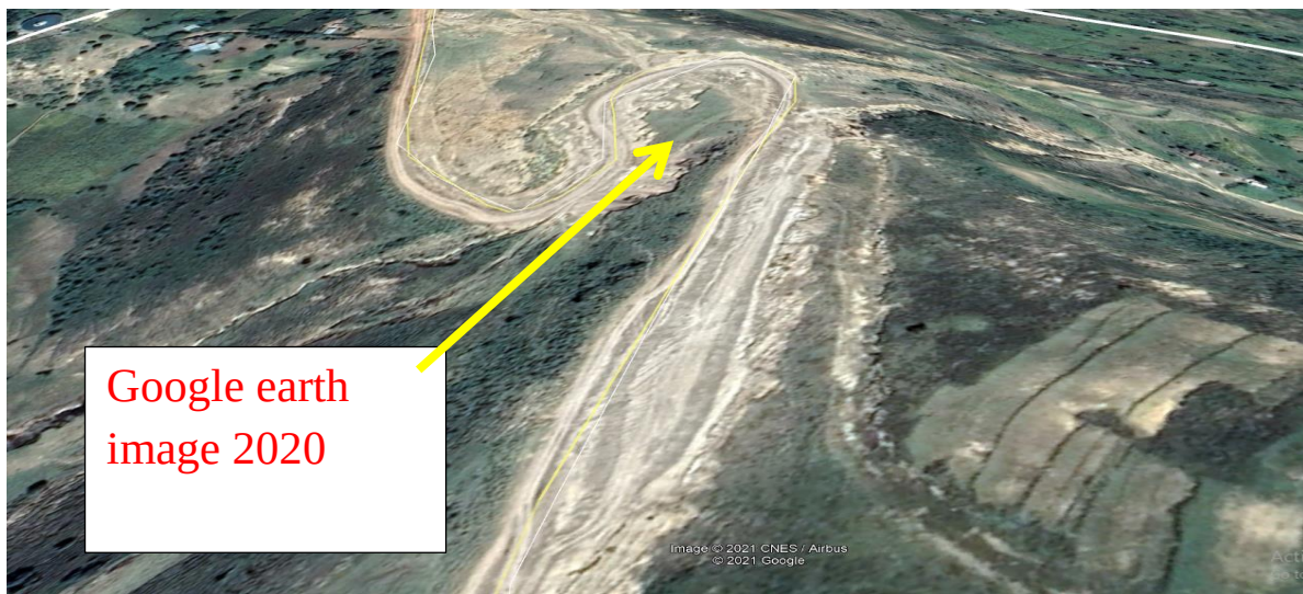
Figure 4.11 (a): Google earth image part of road affected by landslide in 2020
