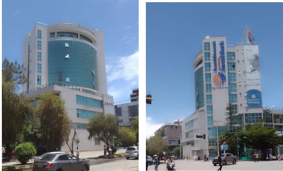
Figure 3.13: Exterior views of Awash bank
