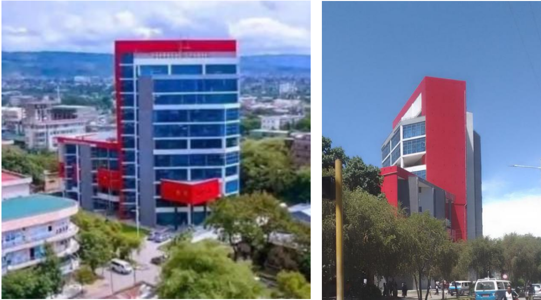
Figure 3.10: Exterior views of Oda building
