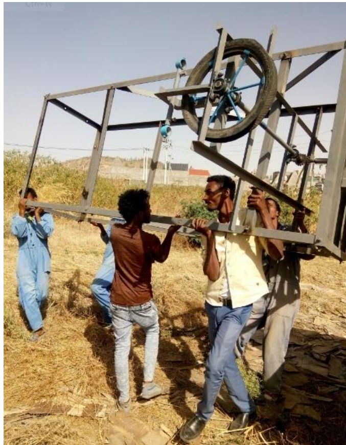
Figure 10. Tower of 3m height used to support the turbine (Photo)
