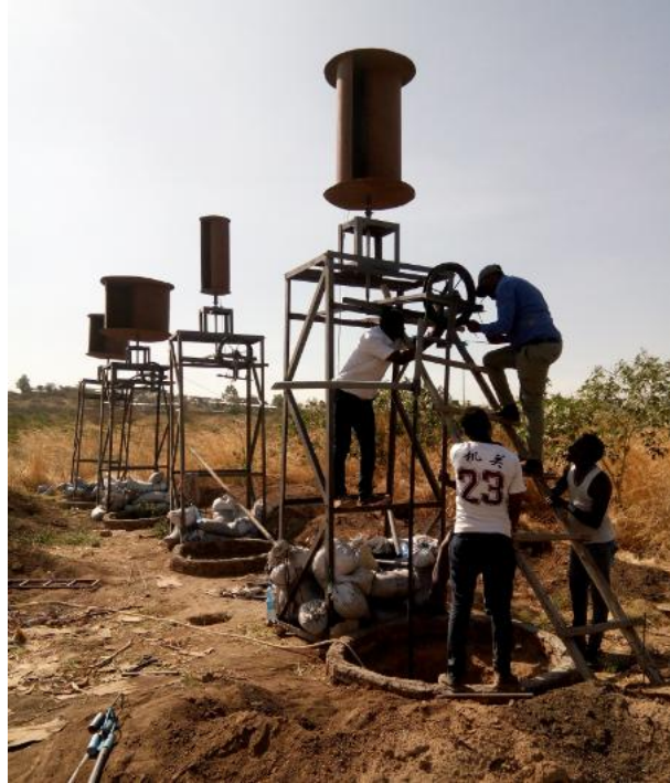
Figure 12. Assembly of the pump and the turbine (photo)
