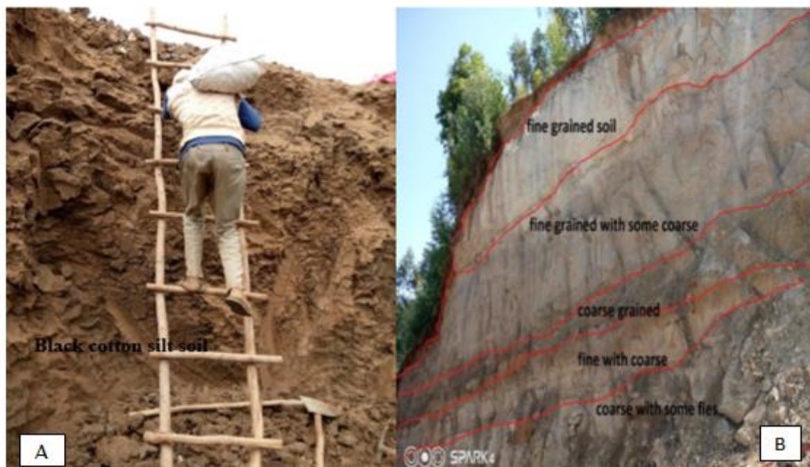
Figure 22: (A) Residual soil deposit from foundation excavation at Hida Kalit Yirgalem agro-industrial Park at GPS reading (long. 429902 m lati.746514 m). (B) Stratified alluvial deposit with rock fragments from the road cut at Arada sub city at GPS reading ( long. 434563 m, lati. 744612 m).
