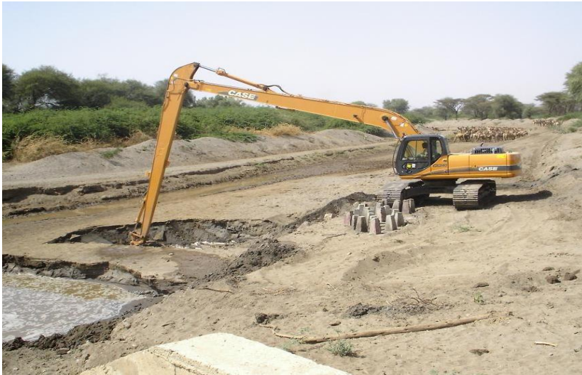
Figure 4.4: Current condition of main canal before disilting
