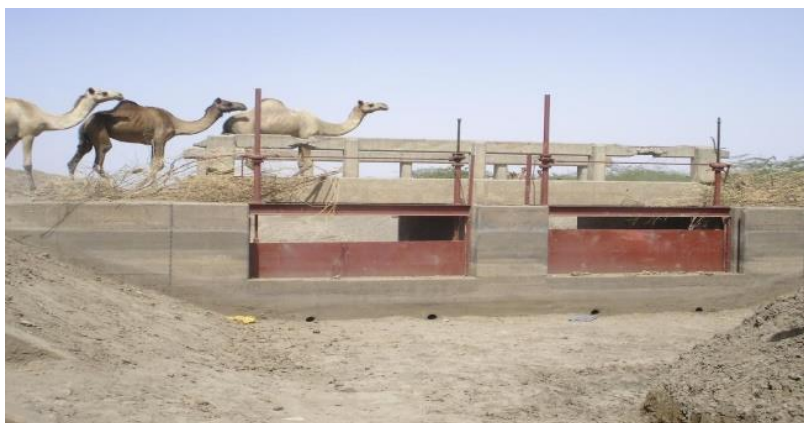
Figure 4.5: Current condition of CD 3
