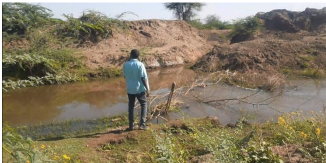
Figure 4.3: Illegal Diversion from main canal (reach CD1-CD2)
