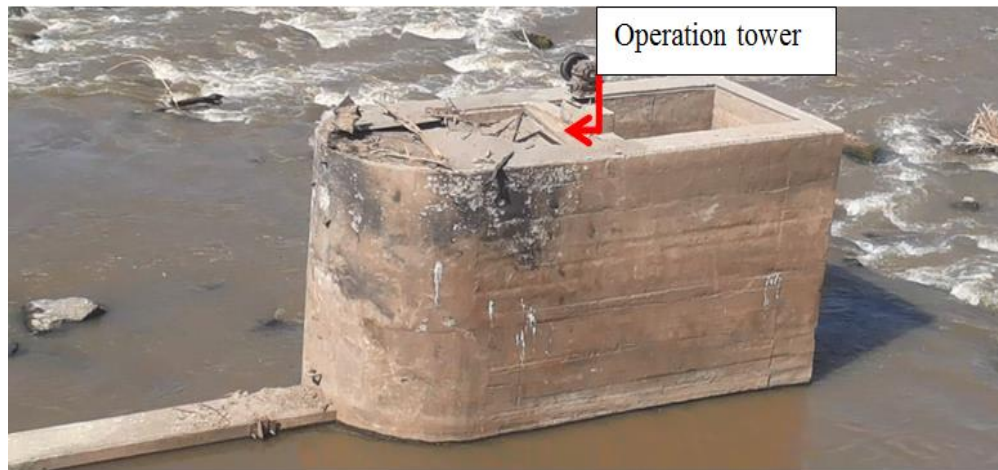
Figure 4.2: Current condition of scouring sluice
