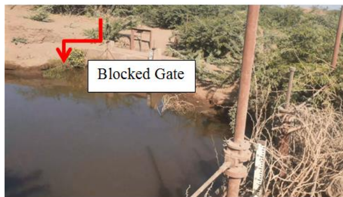
Figure 4.6: Current condition of gated offtake 2 (PO 2 )
