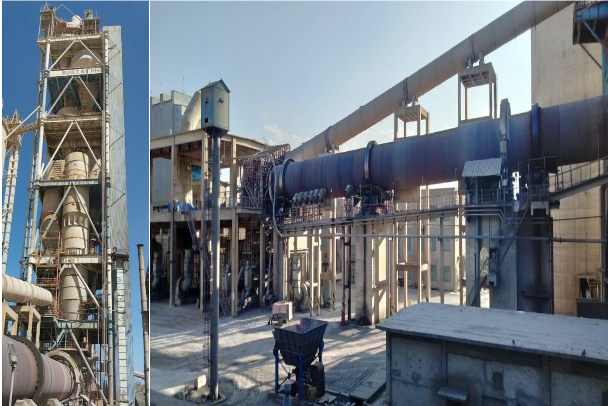
Figure 2.1: National cement 3000 tpd pyro-processing unit
