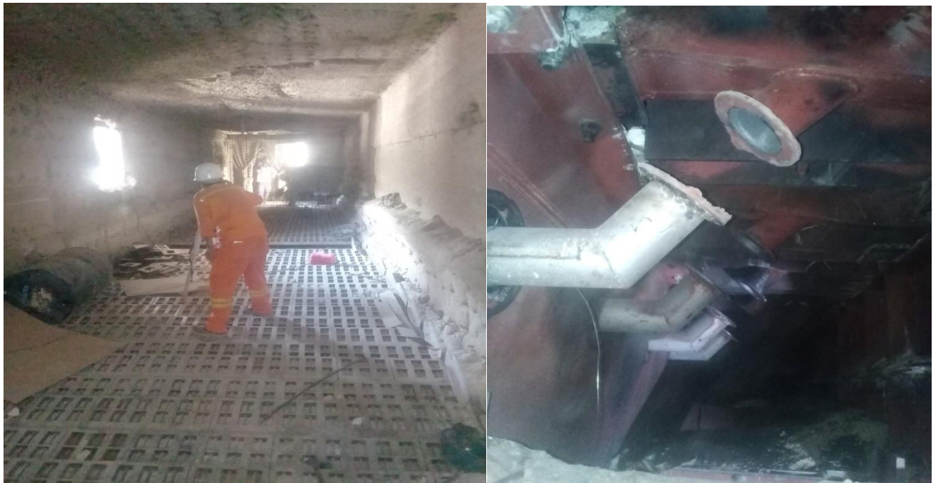
Figure 2.2: NCSC Grate cooler under maintenance on April, 3, 2022
