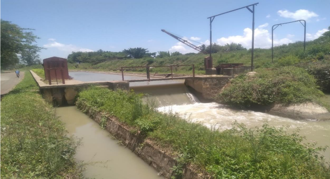
Figure 4.1 Main canal conveyance system at Cipoletti weir
