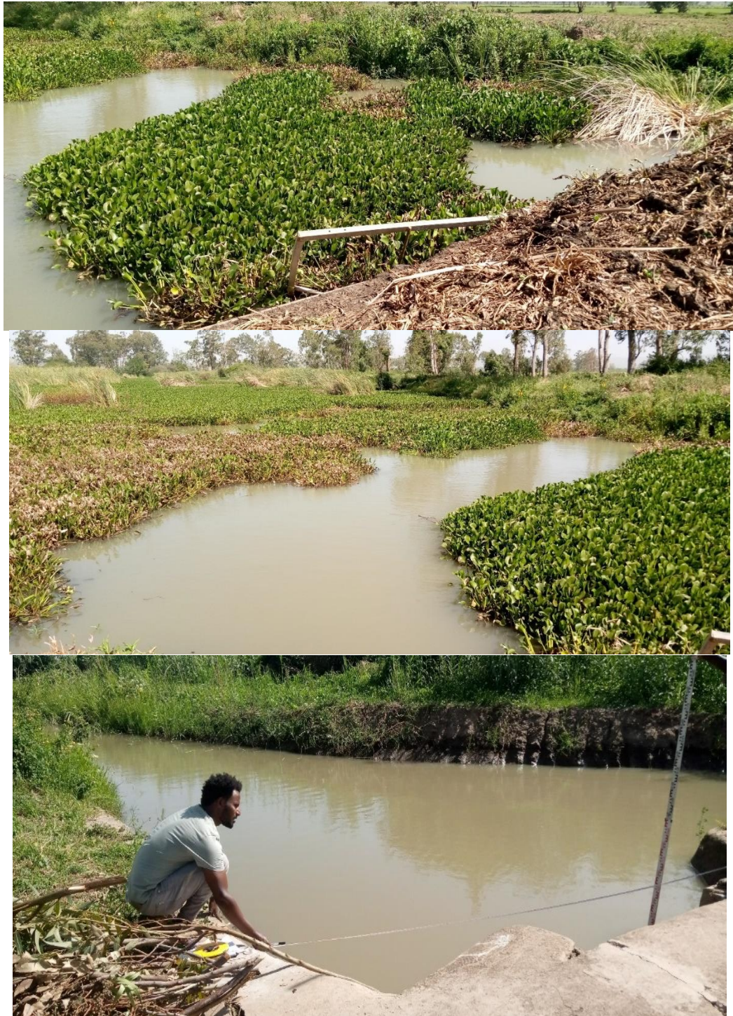
Figure 4.4 Poor management of NSR and inlet of water from left branch canal
