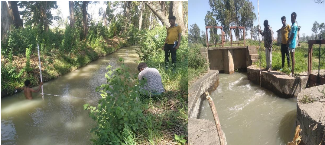
Figure 4.7 Malfunction of canal bank and poor management of division box/offtakes
