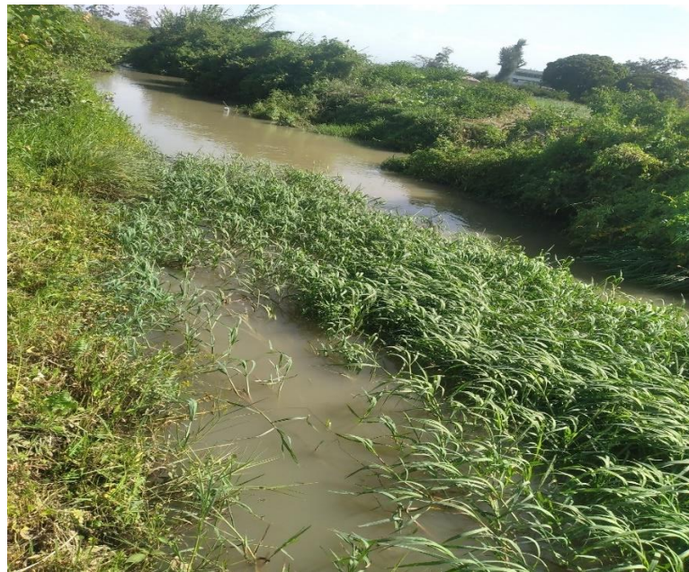
Figure 4.8 vegetation growth at the bank and bed of the secondary canal left branch
