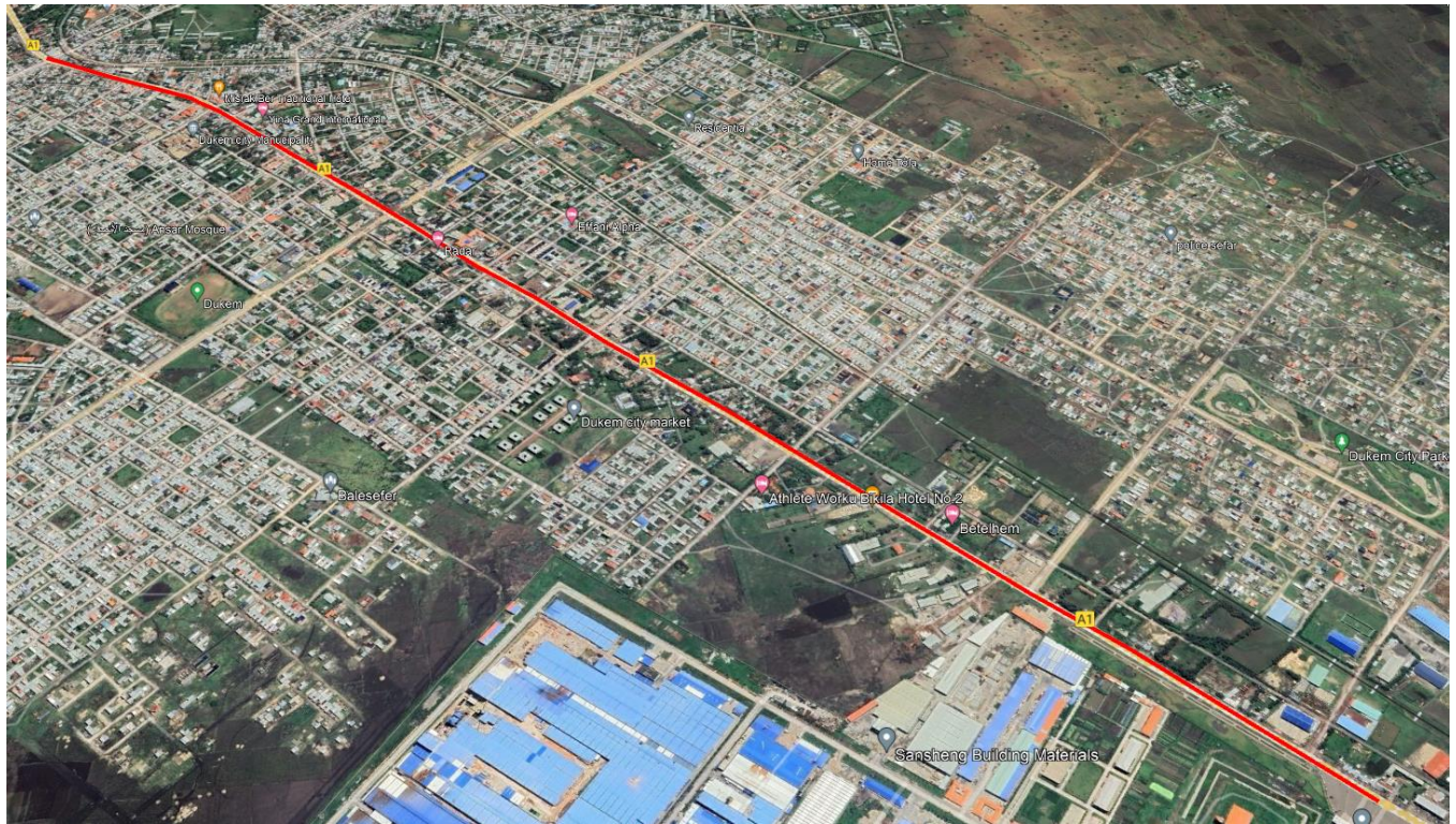
Figure 3:- Main Street of the study area (Addis Kera Asphalt road up to East Industry Zone)
