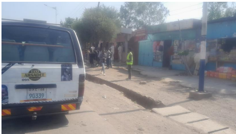
Figure 10: Open ditches in the study area
