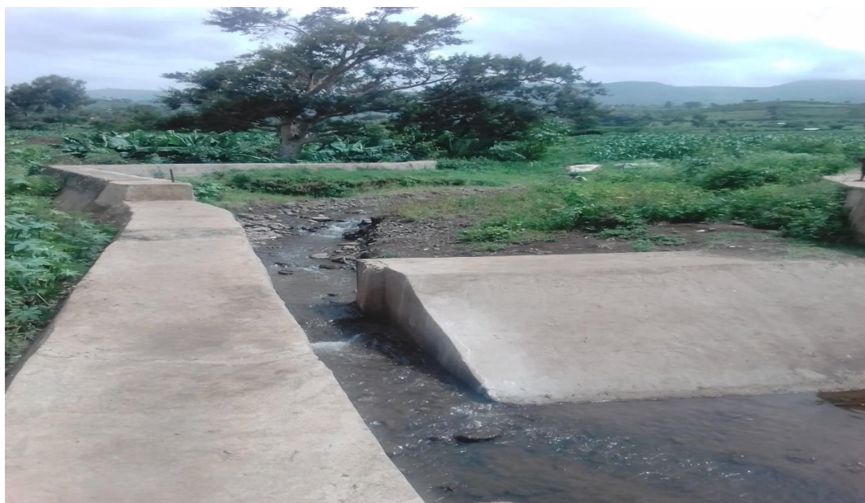
Figure 3.3 Headwork of Jawis irrigation scheme
