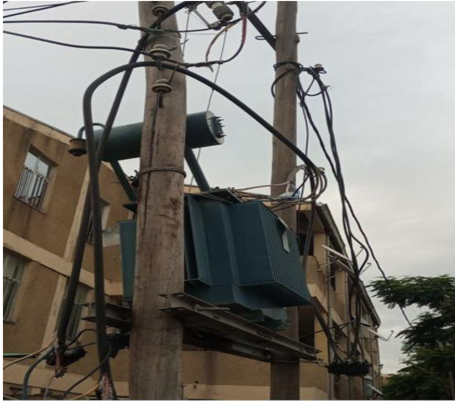
Figure 2. 3 Feeder M-1 aged wooden pole structure on the existing system
