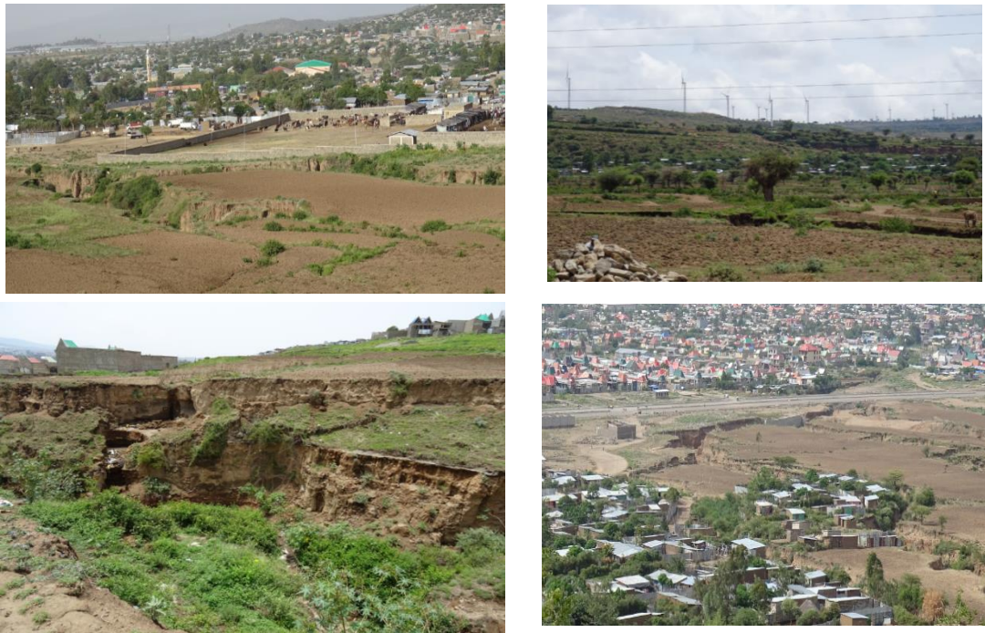
Figure14: Partial view of active gully erosional features in different part of the town
