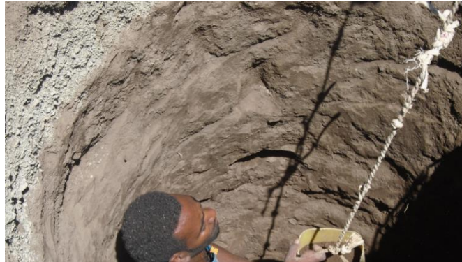
Figure 7: Taking soil sample by digging test pit
